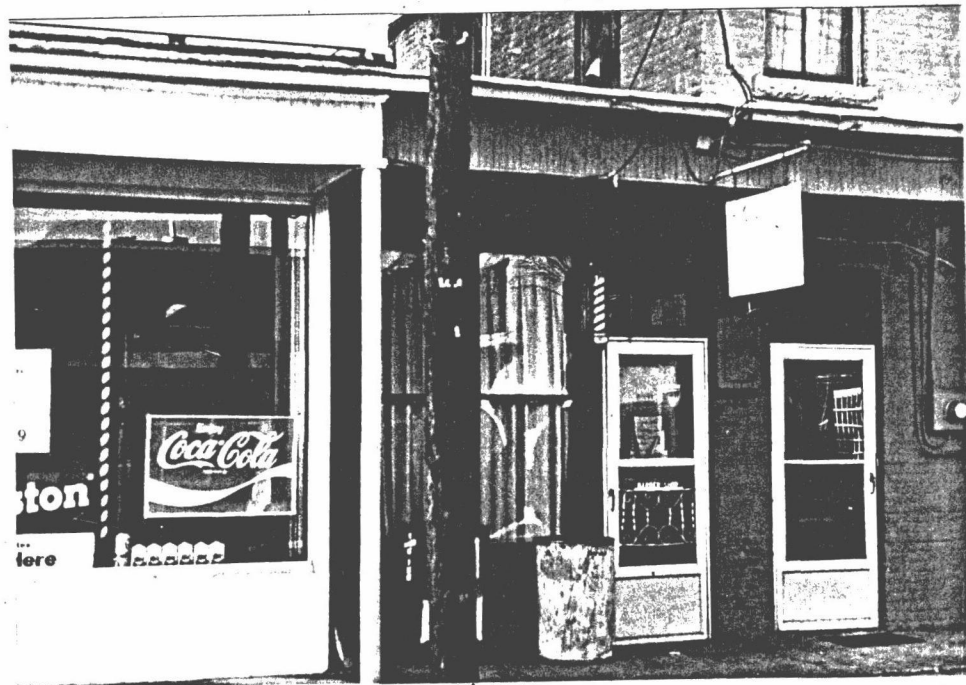
25 241 Main St. 245 Main St.
