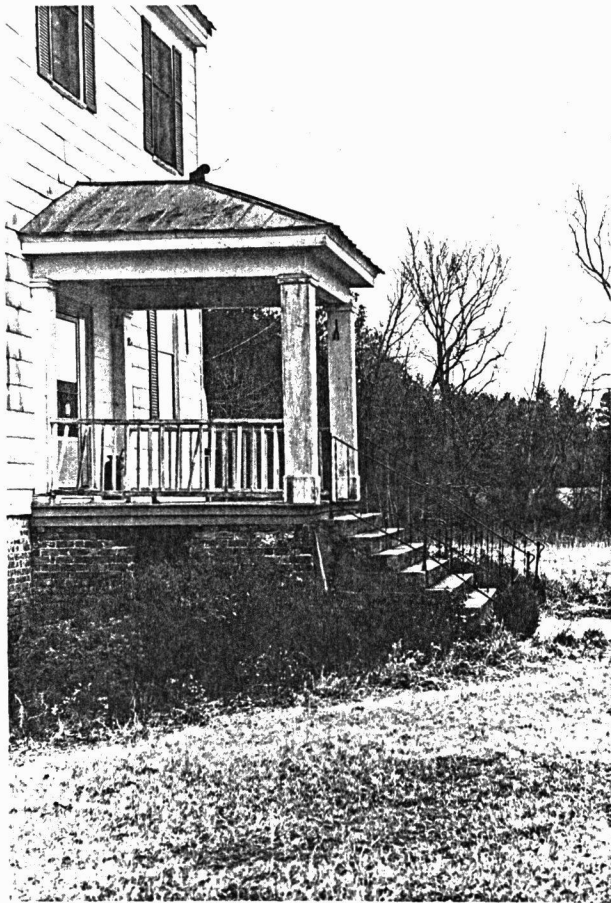
Porch (West Elevation)
