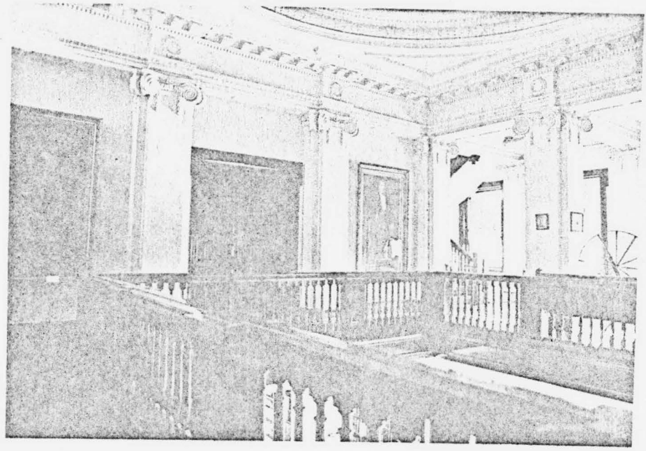
Second floor, mezzanine
