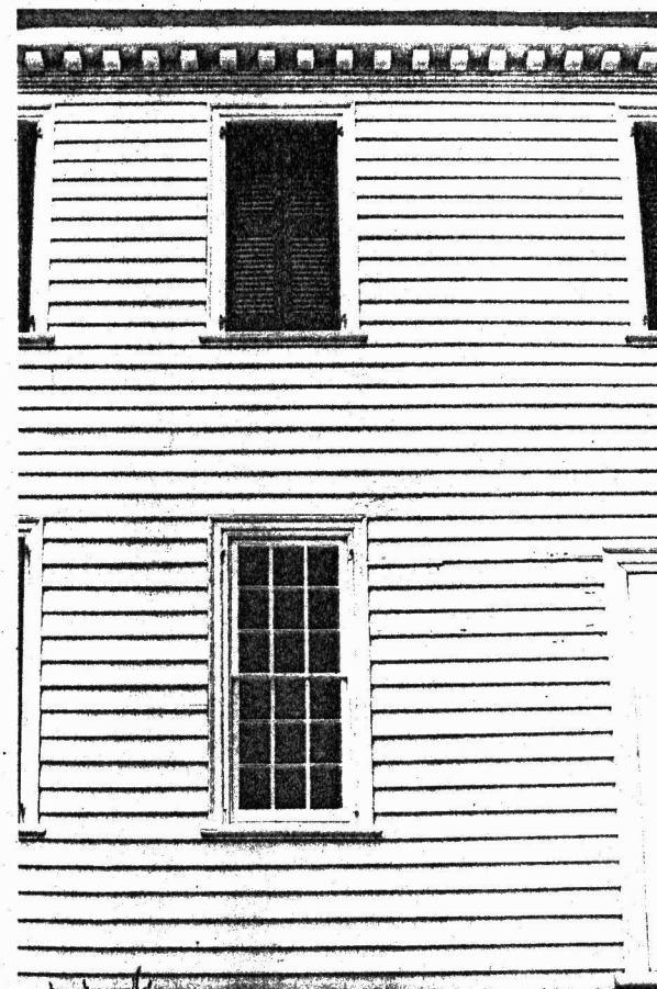
Detail of dentil cornice & weatherboarding
