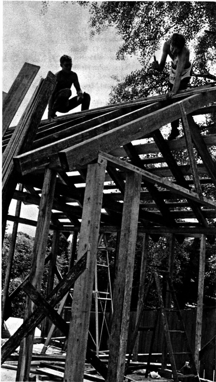
Builders reconstructing Jackson's carriage house employed 19th century building techniques.
