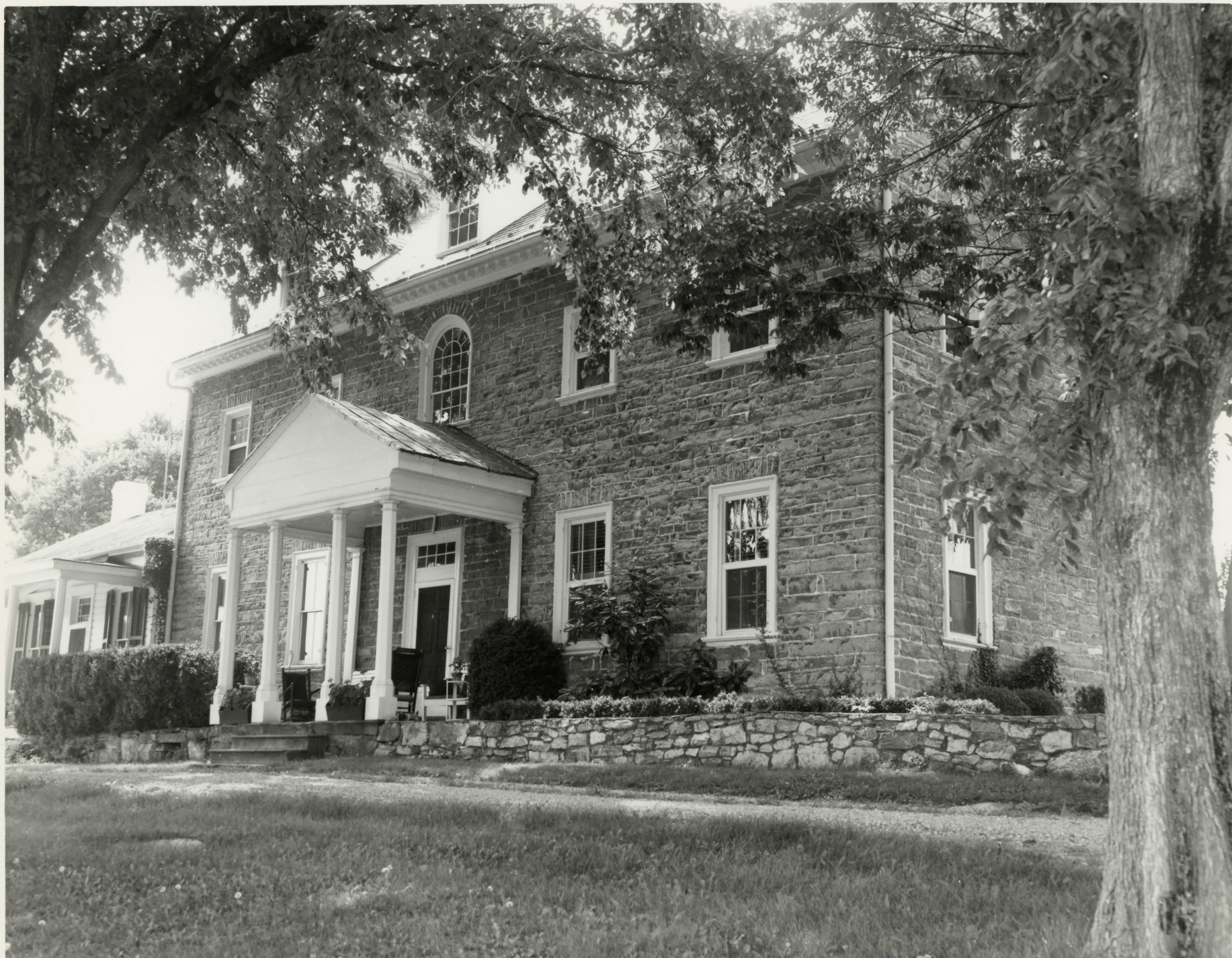
General Daniel Morgan House, Saratoga, Boyce, Virginia. (South elevation).
