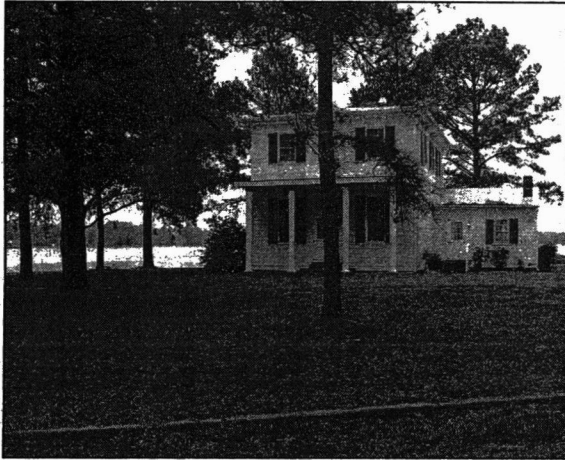
The former B. Williams and Co. Store at Williams Wharf will be preserved, thanks to a $345,000 grant from the Virginia Land Conservation Foundation.
