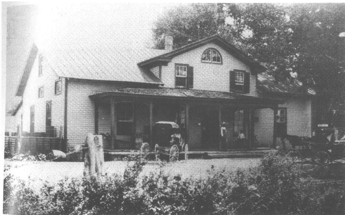
Figure 5. 1914 photograph of the south façade of the Ware Neck Store and Post Office (Sinclair 1991:77).
