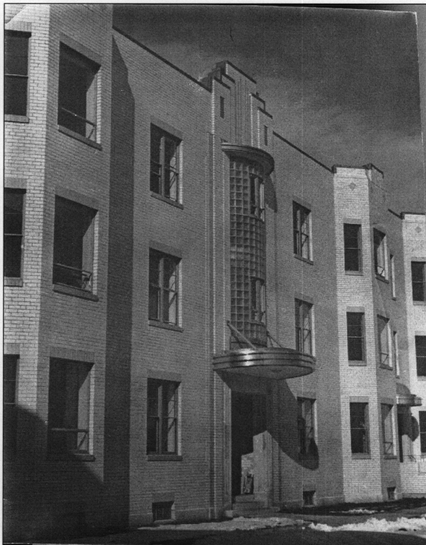
Figure 2 Historical photo of Rosedale Apartments Rear elevation, ca 1940 Courtesy of Steven R. and Joanna Hunt
