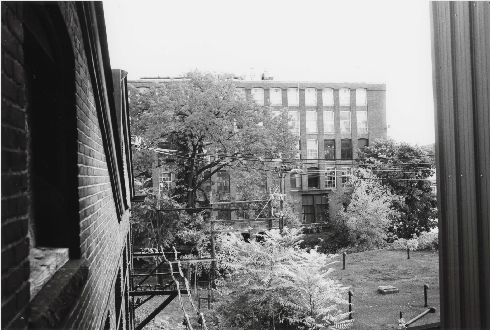
NORTH ELEVATION of FINISHING BUILDING GREYSTONE MILL HISTORIC DISTRICT NORTH PROVIDENCE, PROVIDENCE COUNTY RHODE ISLAND PHOTOGRAPH NUMBER 11
