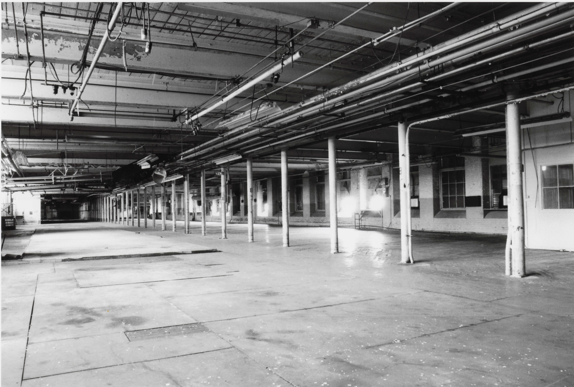
INTERIOR VIEW of MAIN MILL GREYSTONE MILL HISTORIC DISTRICT NORTH PROVIDENCE, PROVIDENCE COUNTY Rhode Island PHOTOGRAPH NUMBER 14
