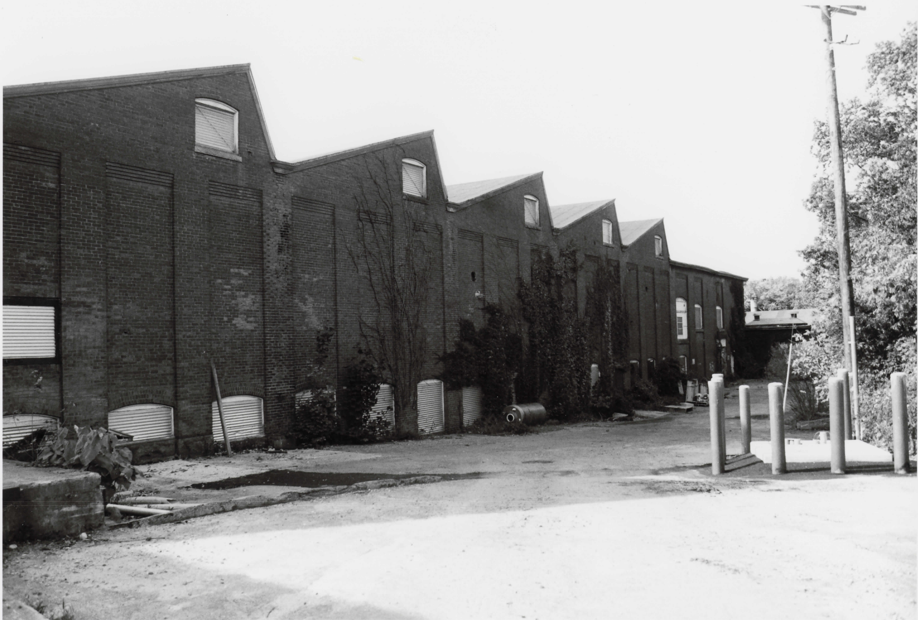
DYE HOUSE WITH WEAVE SHED AT RIGHT GREYSTONE MILL HISTORIC DISTRICT NORTH PROVIDENCE, PROVIDENCE COUNTY RHODE ISLAND PHOTOGRAPH NUMBER 6
