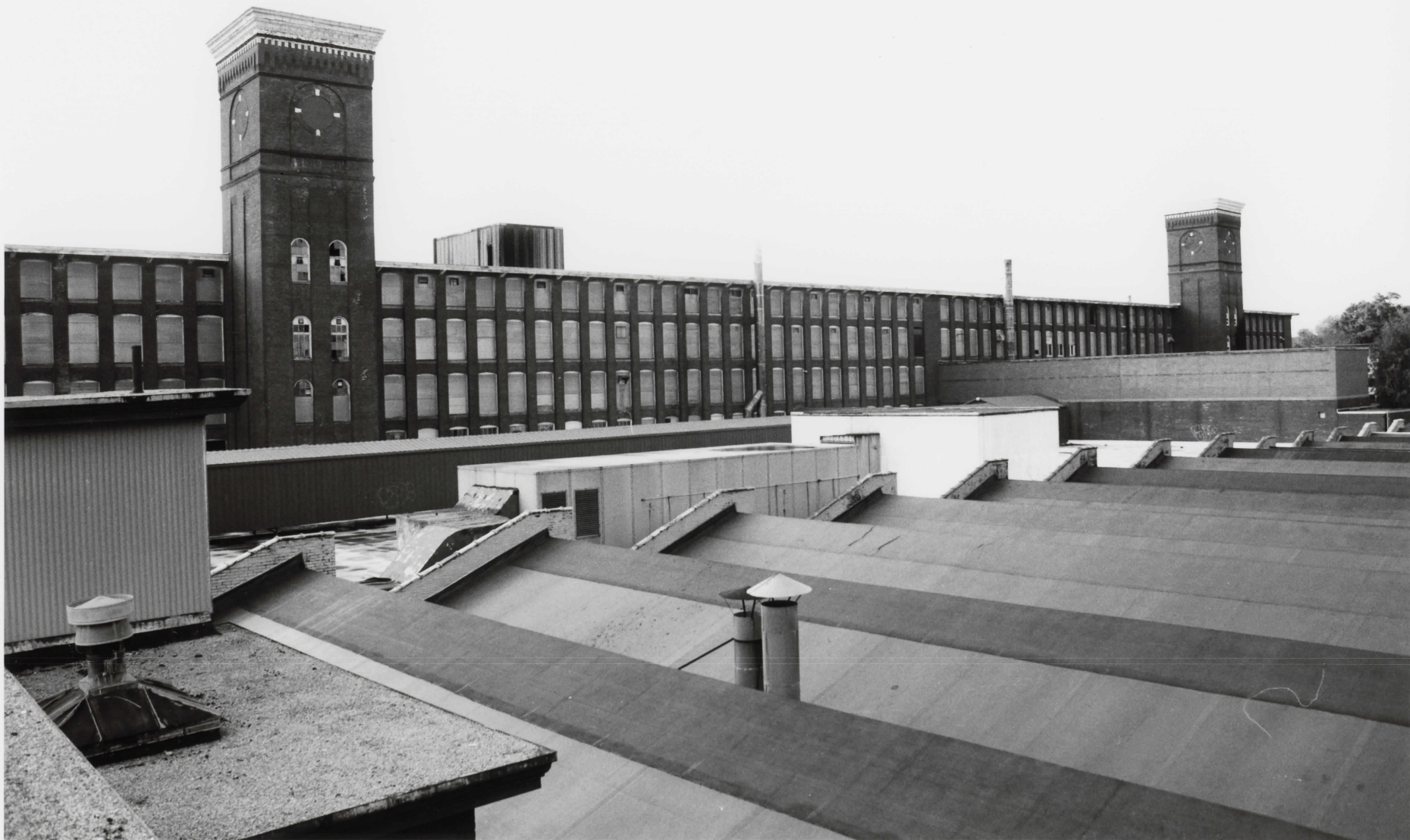
WEAVE SHED AND MAIN MILL GREYSTONE HISTORIC DISTRICT NORTH PROVIDENCE, PROVIDENCE COUNTY Rhode Island PHOTOGRAPH NUMBER 5
