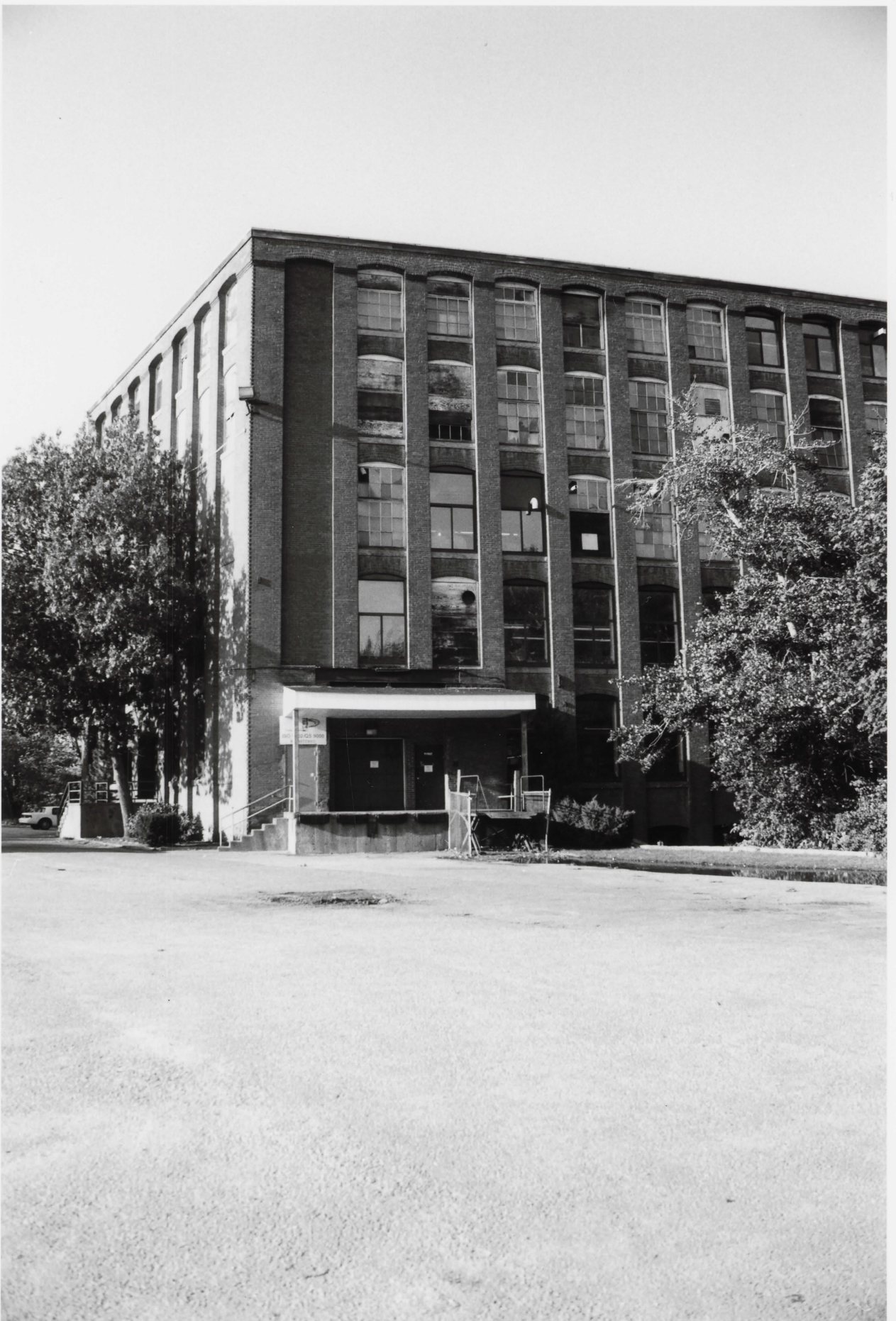
WEST END OF FINISHING BUILDING GREYSTONE MILL HISTORIC DISTRICT NORTH PROVIDENCE, PROVIDENCE COUNTY RHODES ISLAND PHOTOGRAPH NUMBER 8
