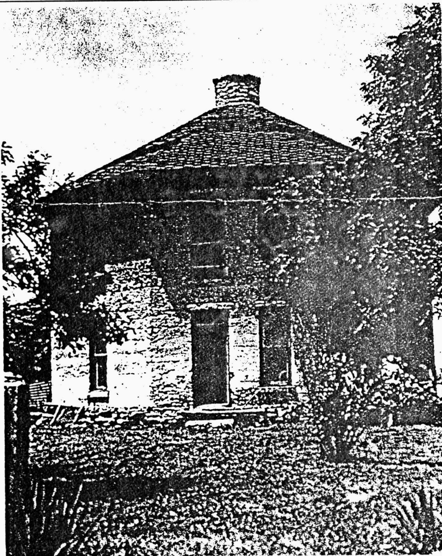
This photo is of the Cole House in 1936, when Ed West owned the property. This photo was placed on postcards and sold in the nearby city of Houston, Texas County.
