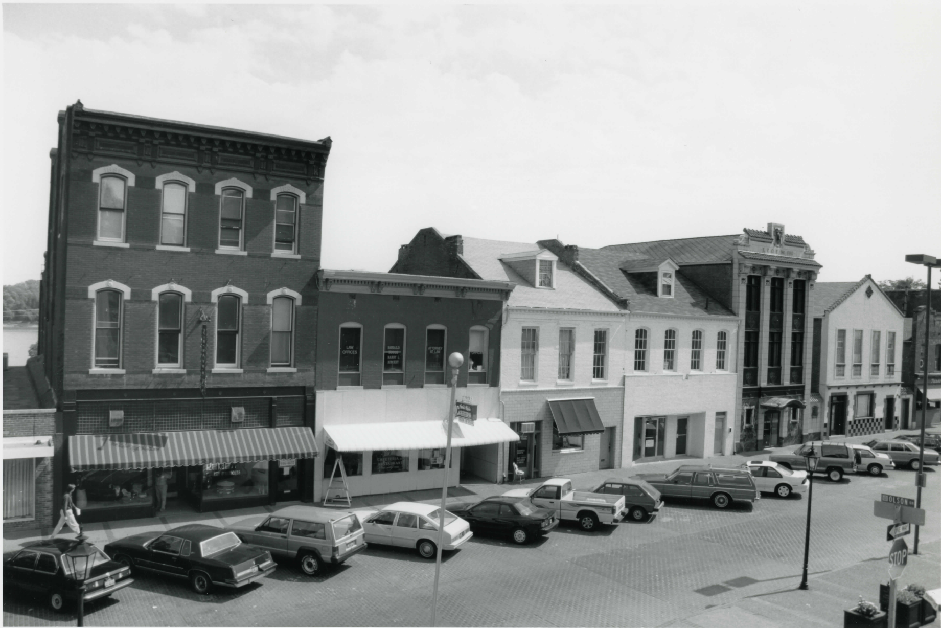
2 EAST SIDE 100 BLOCK S. MAIN 104, LEFT CAMERA FACING SOUTHEAST
