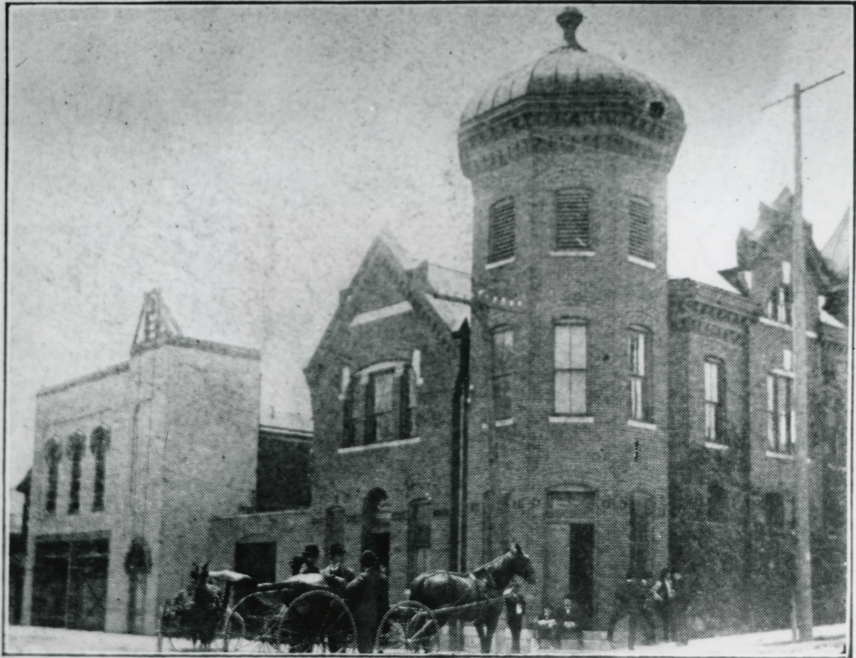
CITY HALL AND FIRE HEADQUARTERS.
