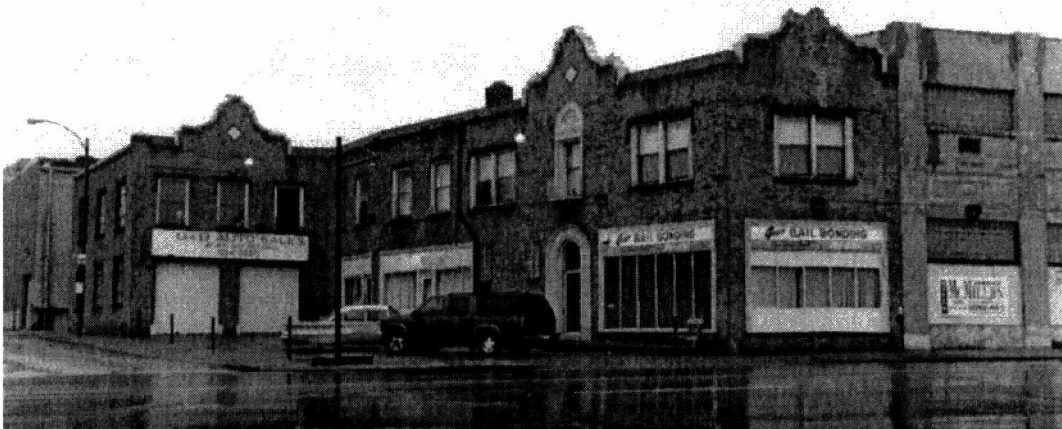
Becker-Lehman Sales Company Building, (Tire Company) 3043 Olive
