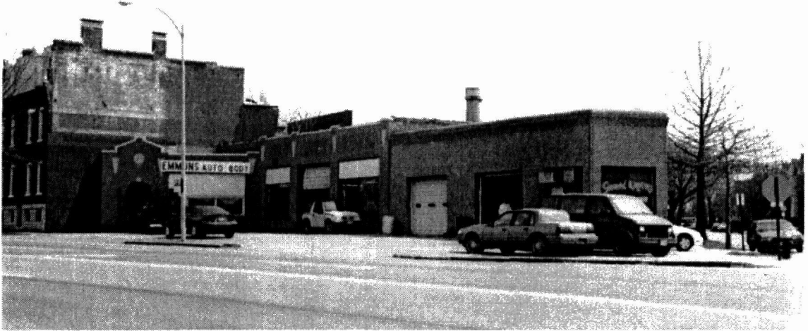
Service Garage 2230 Gravois
