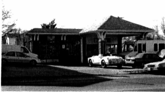
Gas Station 6300 Block of Arsenal
