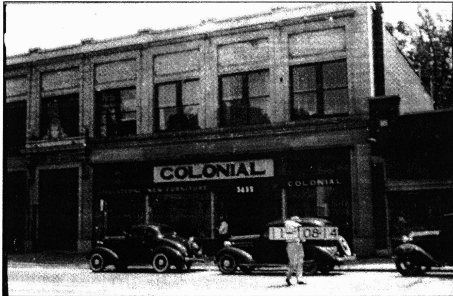
Figure 7 South end of Main Façade facing northeast Photos: Insurance photographs from the 1940s. Courtesy of the Landmarks Commission, Kansas City, Missouri.
