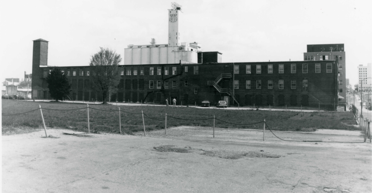
D.M. Oberman Mfg. Co. 600 Bonville Avenue Springfield, Greene Co., MO Photo 8
