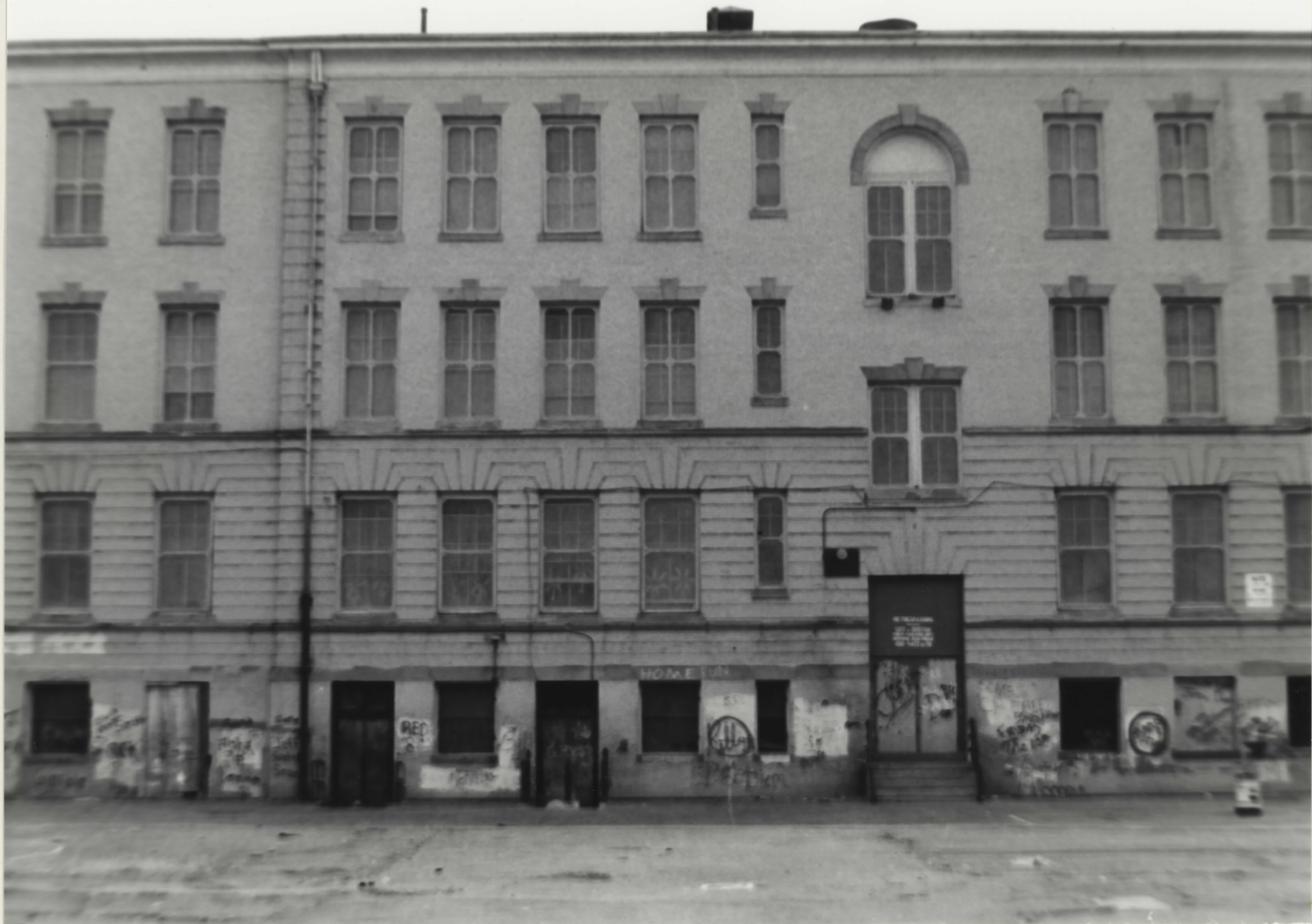
WESTERLY FACADE AND ENTRANCE (Existing Parking Lot Side)
