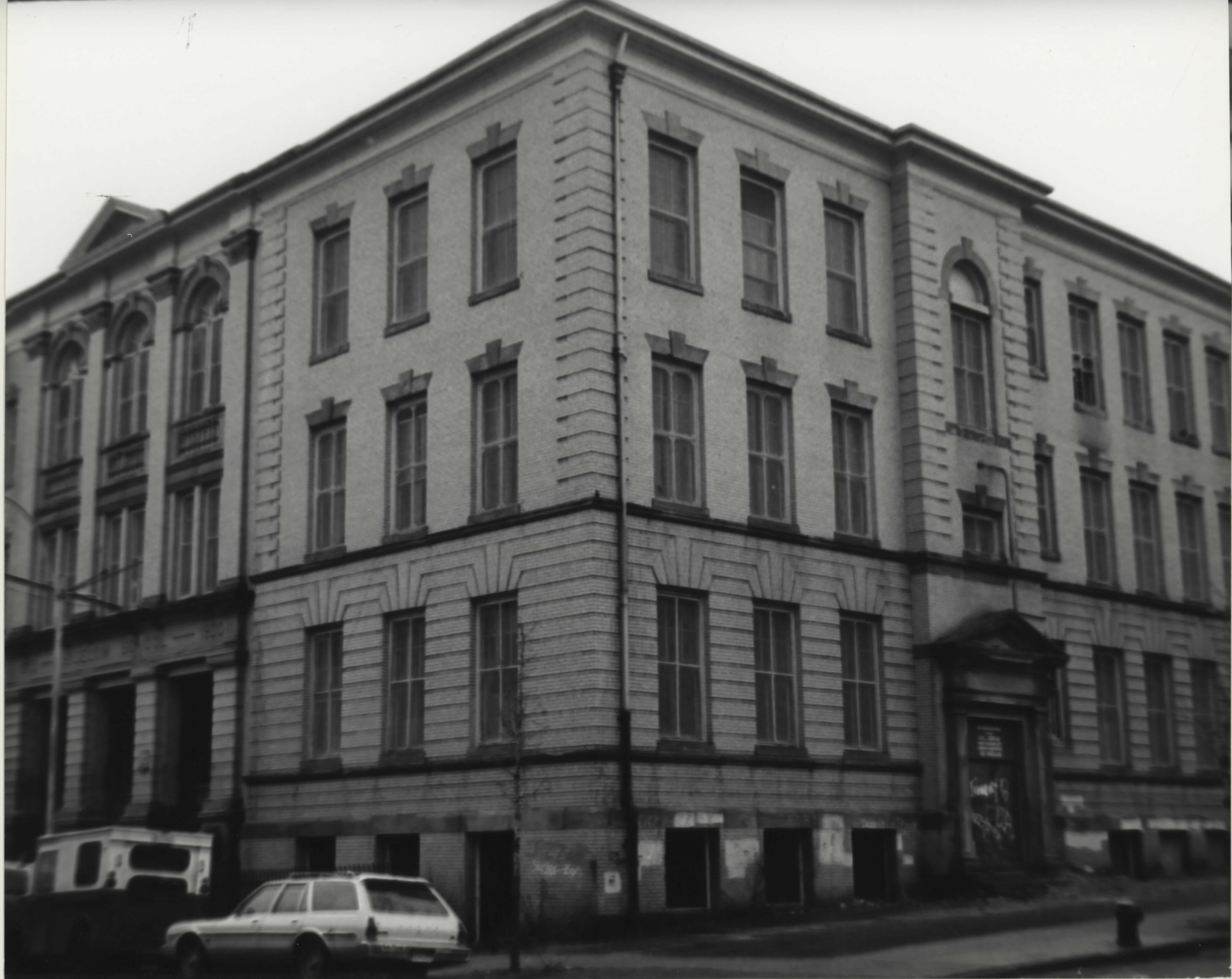
BUILDING FRONT AND EASTERLY SIDE (Corner of E & 4th)
