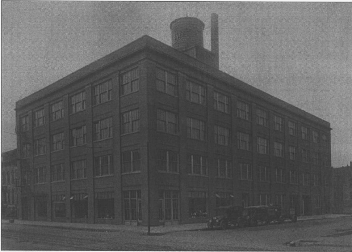
Figure 1: Vesta Accumulator Company Building, 1910 (Photograph courtesy of Chicago Historical Museum)
