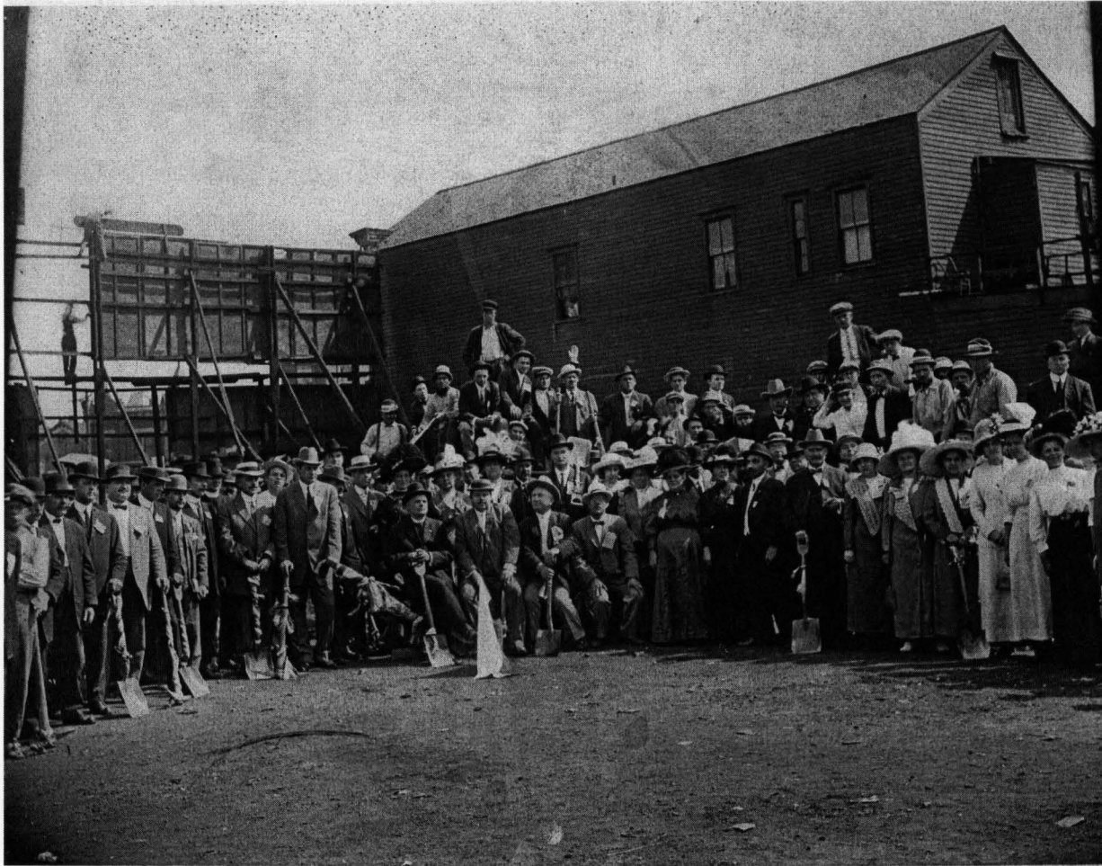
Polish Roman Catholic Union Building Ground breaking in 1912, facing unknown
