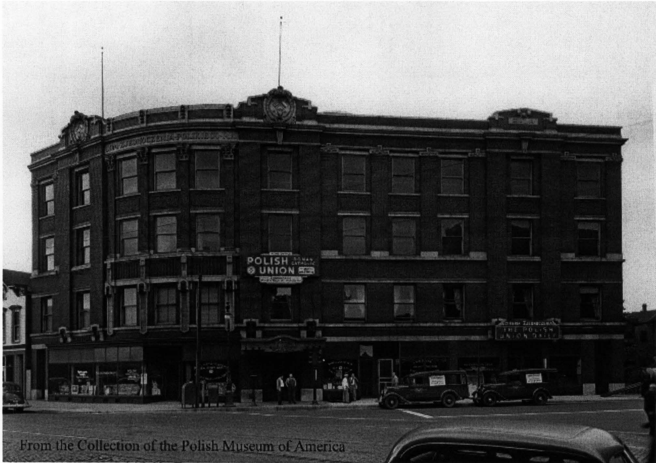
Polish Roman Catholic Union Building_ North and northeast facade in 1913
