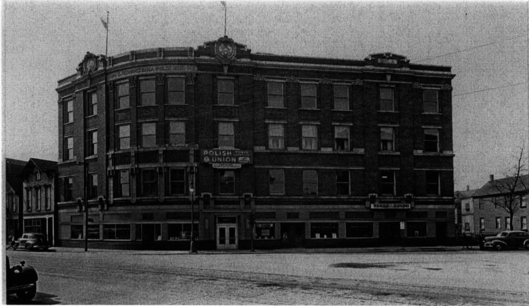
Polish Roman Catholic Union Building_ North and northeast facade in 1941
