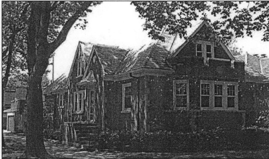
Figure 19: 6500 North Talman Avenue
