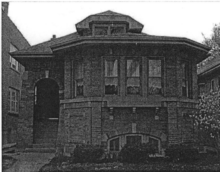
Figure 25: 6724 North Talman Avenue
