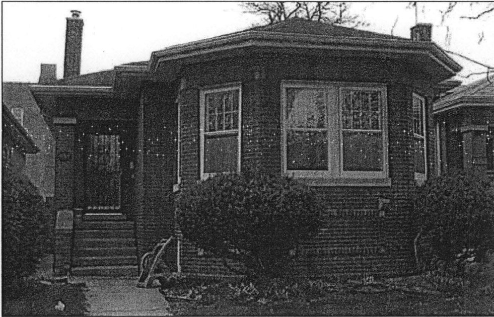
Figure 26: 6704 North Talman Avenue
