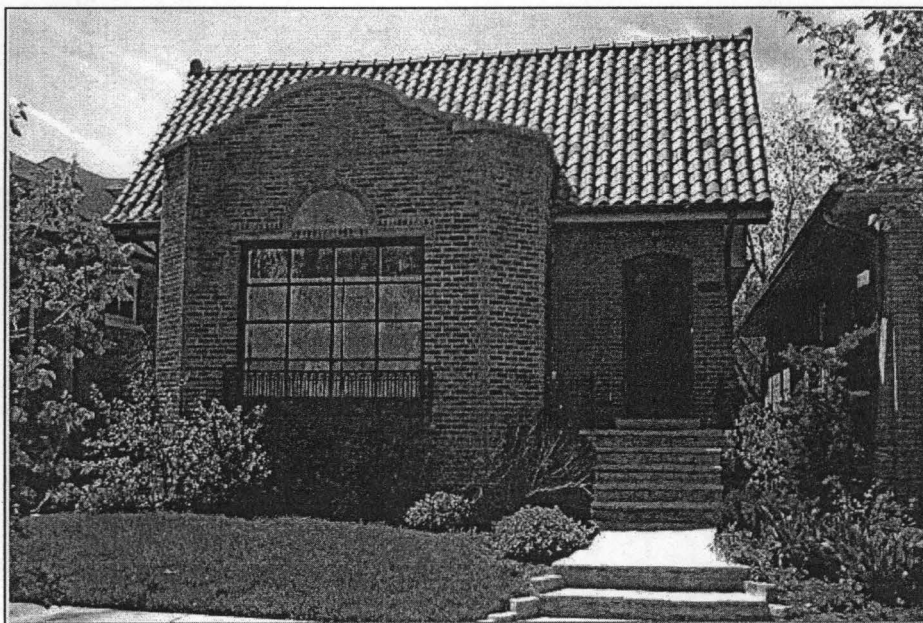
Figure 16: 6554 North Talman Avenue
