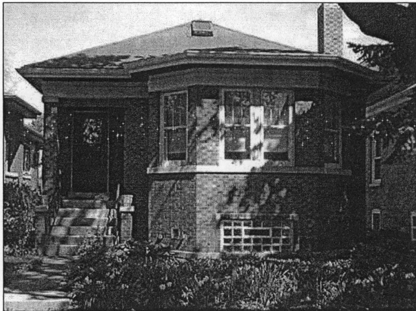
Figure 11: 6511 North Talman Avenue
