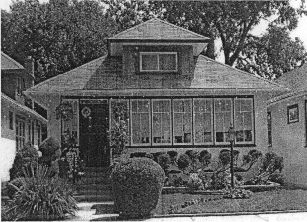
Figure 1: 7641 South Merrill Avenue
