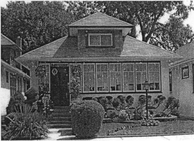
Figure 1: 7641 South Merrill Avenue
