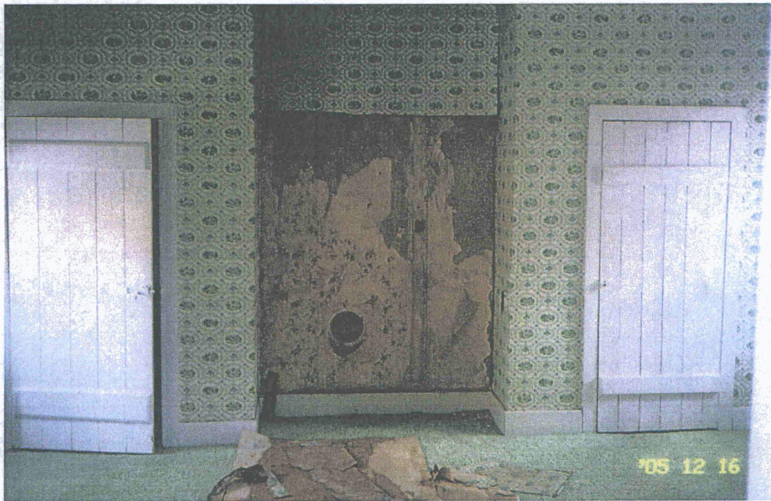
IL_MorganCounty_Woodlawn14 Interior. East bedroom, second floor, showing added closets of 1928 with 20 th century board/batten doors. Camera facing east.
