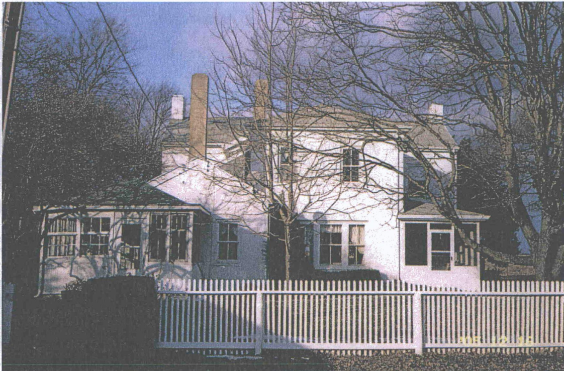
IL_MorganCounty_Woodlawn04 South Elevation. Camera facing north.
