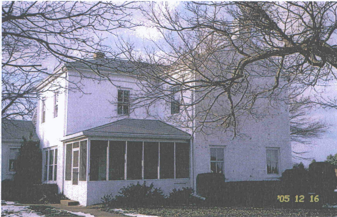
IL_MorganCounty_Woodlawn03 East Elevation. Camera facing northwest.
