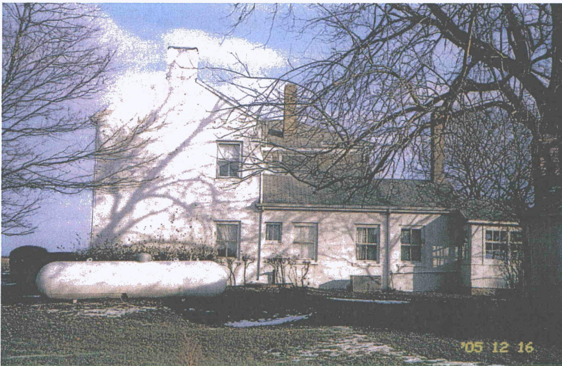
IL_MorganCounty_Woodlawn05 West Elevation. Camera facing east.
