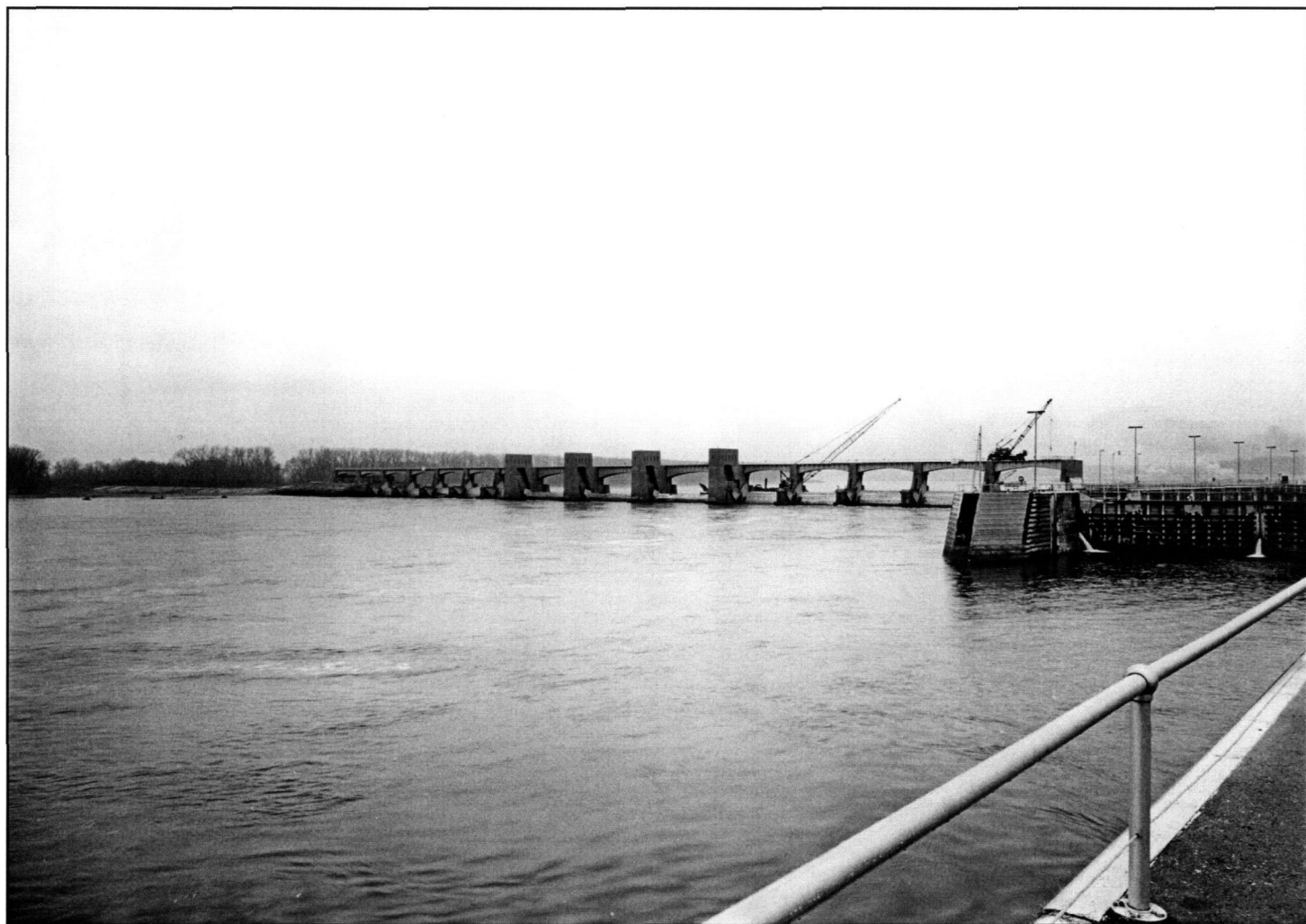
PHOTO 3. General View of Dam, Downstream Side. Photographer: Peter A. Rathbun Date of Photograph: September 1987 Location of Original Negative: IL-30-2, HAER, IL, 1-QUI, 5- HAER Collection, Prints and Photographs Division, Library of Congress, Washington, D.C. View: From downstream guide wall of main lock looking north
