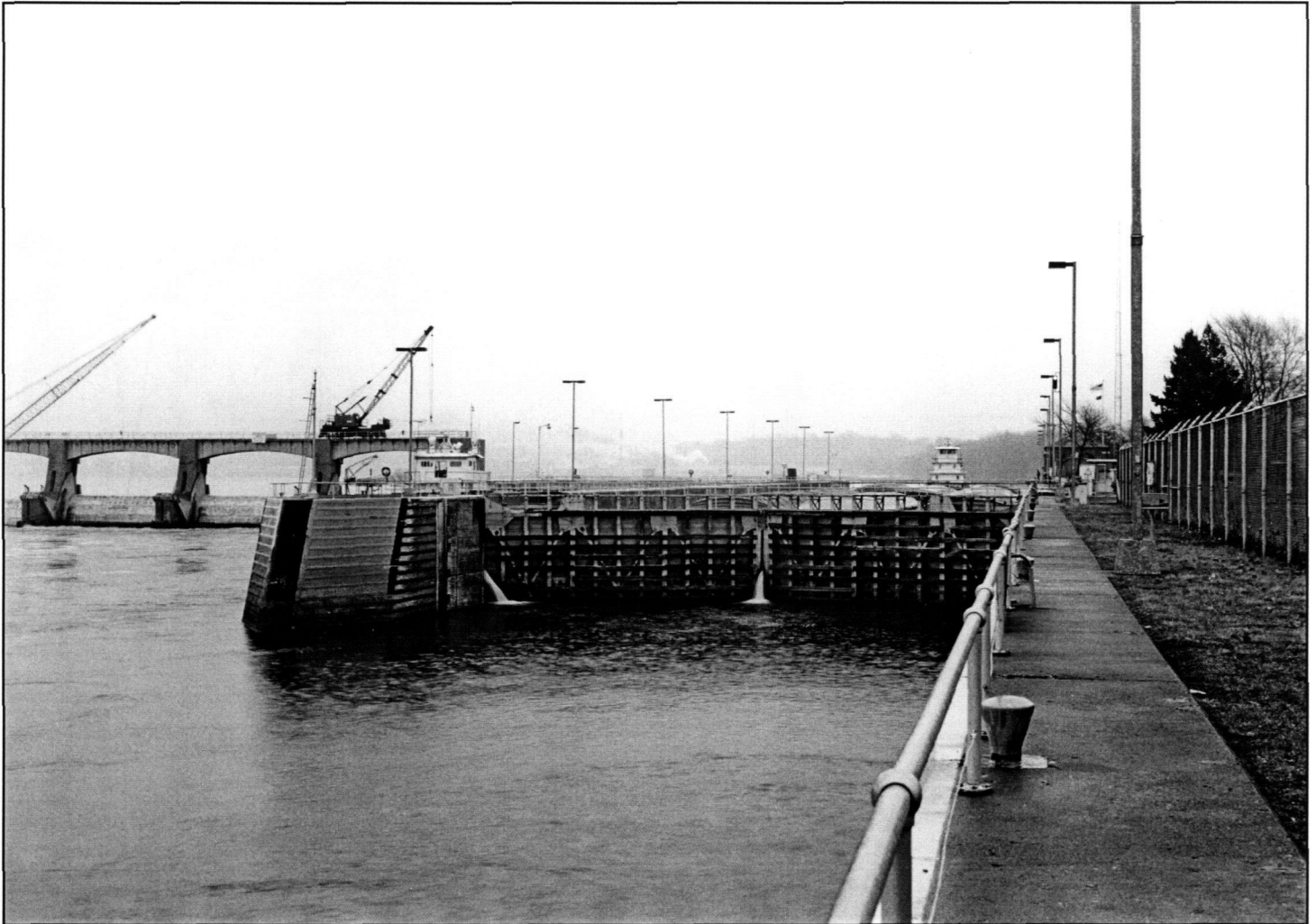
PHOTO 2. General View of Main Lock, Downstream Side. Photographer: Peter A. Rathbun Date of Photograph: September 1987 Location of Original Negative: IL-30-3, HAER, IL, 1-QUI, 5- HAER Collection, Prints and Photographs Division, Library of Congress, Washington, D.C. View: From downstream guide wall of the main lock, looking northeast
