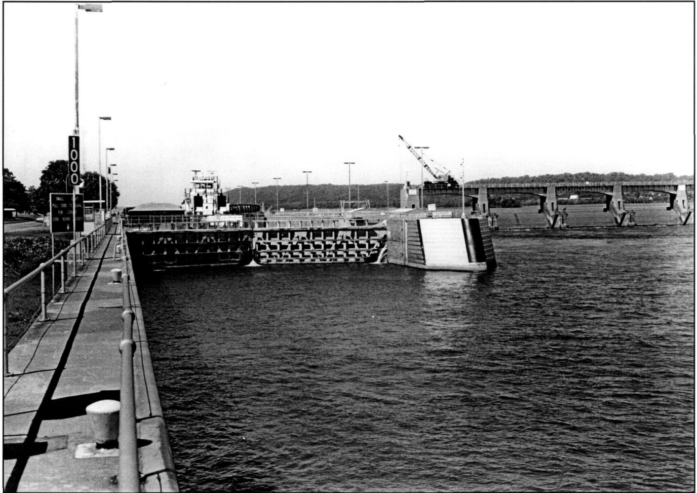
PHOTO 2. General View of Lock, Downstream Side.
