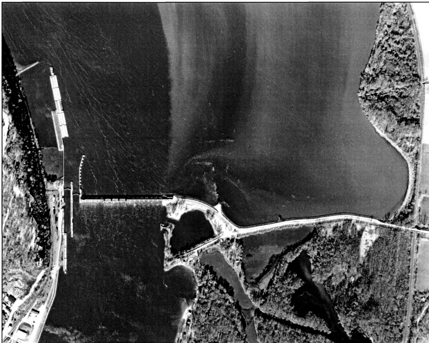
PHOTO 1. Aerial Photo of Lock and Dam No. 11.
