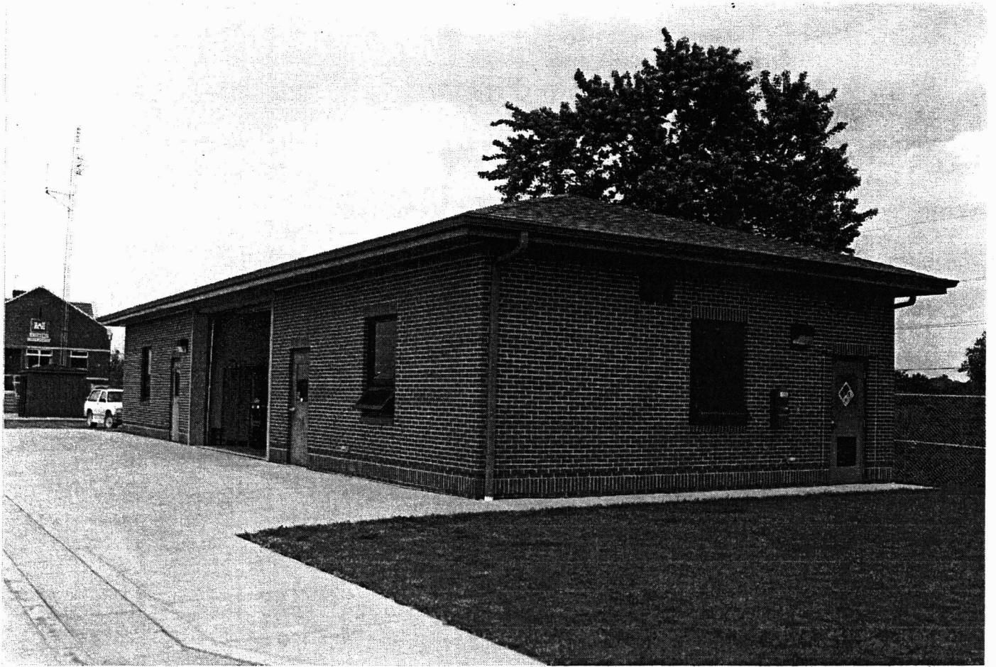
Figure 7. Maintenance building to northeast, Lockport Lock, Dam, and Power House Historic District, Will County, Illinois (Photographed by B. J. Henning 2001).
