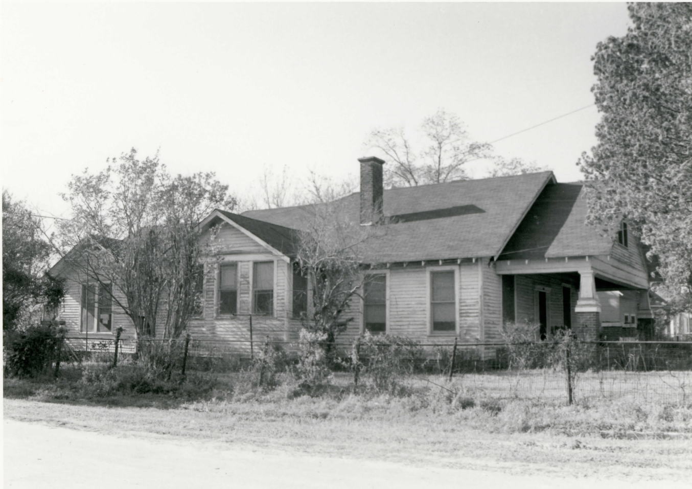
CL-49 Anderson Boarding House 201 Main HISTORIC RESOURCES OF CLARENDON Jeff Lewellen, photographer Negatives at AHPP Viewed from the Southeast
