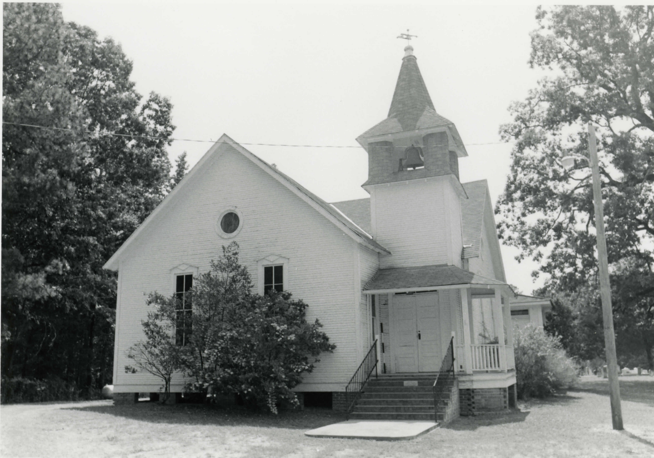
DA-22 Sardis Methodist Church Don Brown, photographer May 18, 1982 Negative filed at the AHPP View from the West
