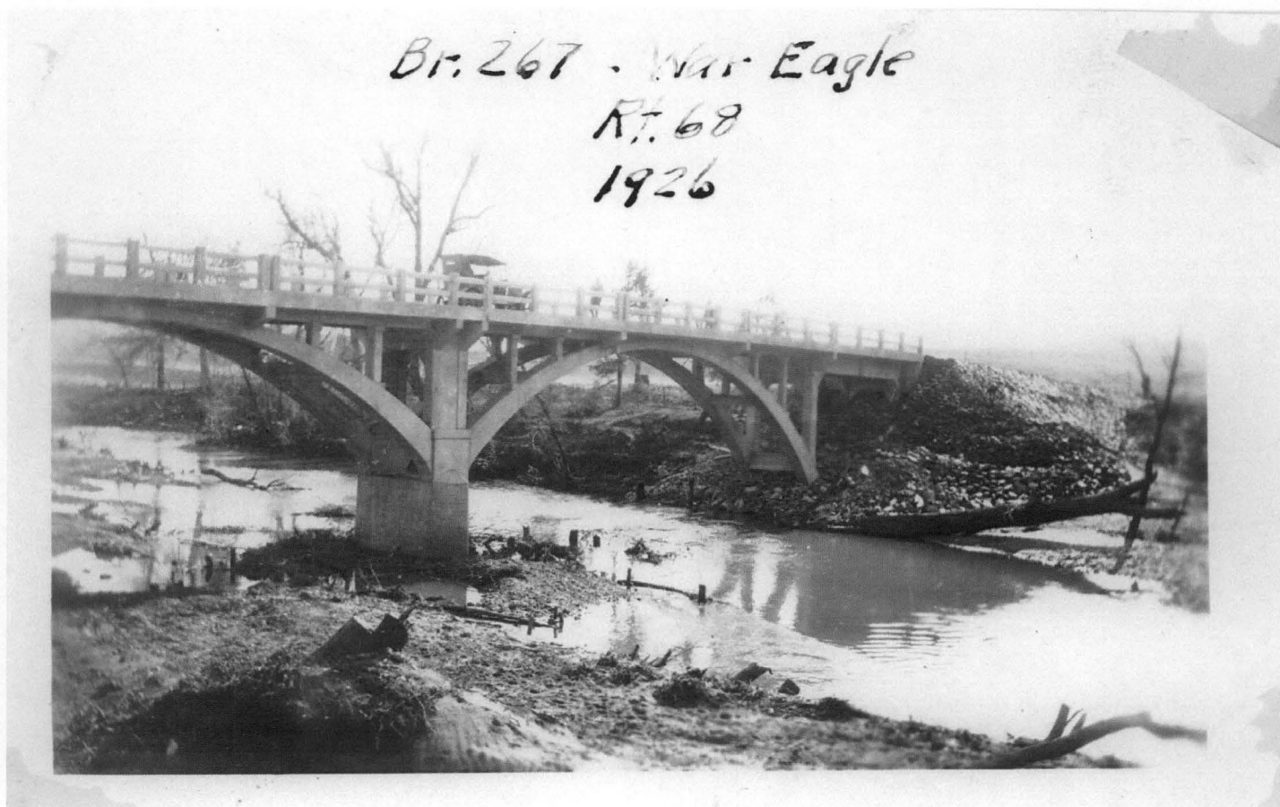
1926 picture of the War Eagle Creek Bridge
