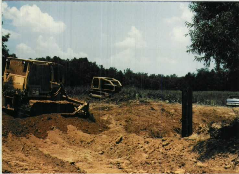
Fig. 15. A field impoundment nears completion adjacent to the Auxiliary Channel. Six impoundments were constructed in Little Twist Field this summer. 09/87 DME
