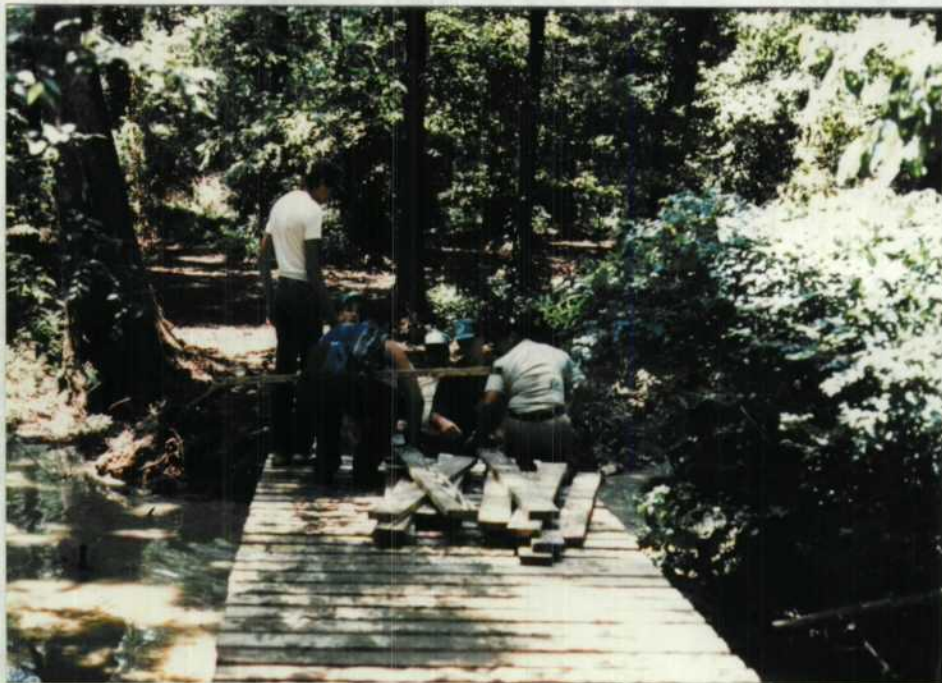
Fig. 13. A 70-foot ATV bridge was constructed as part of a new trail south of Brushy Lake. YCC workers from Yazoo NWR assisted Panther's staff and YCC with this project. 07/87 DME
