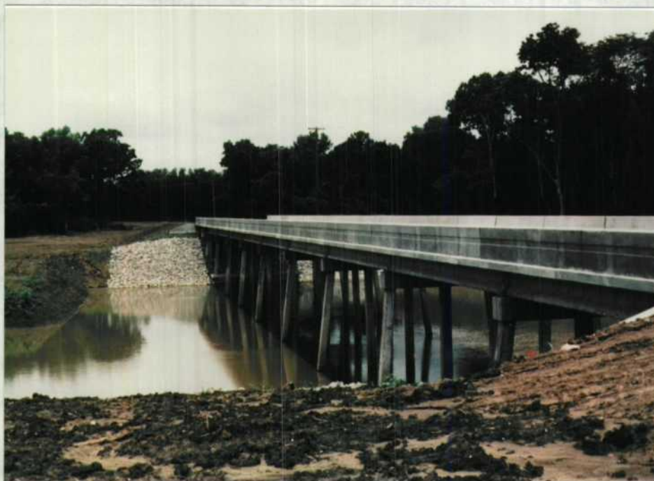
Fig. 30. A new bridge was constructed at Bear Garden to accommodate the widening of Steele Bayou by the U.S. Army Corps of Engineers.
