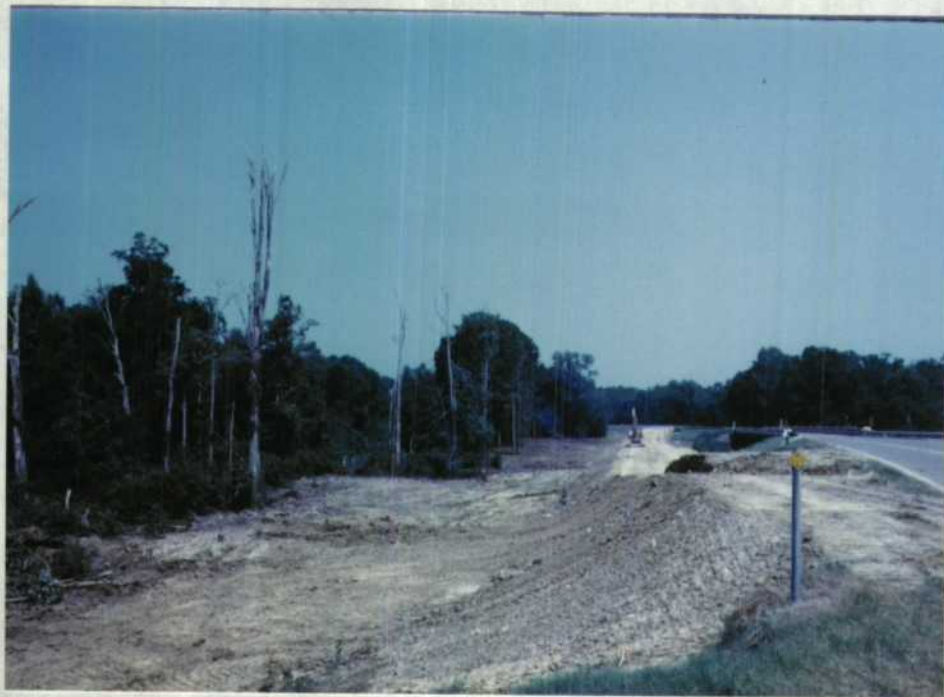
Fig. 2. Highway Construction 08/87 HWB
