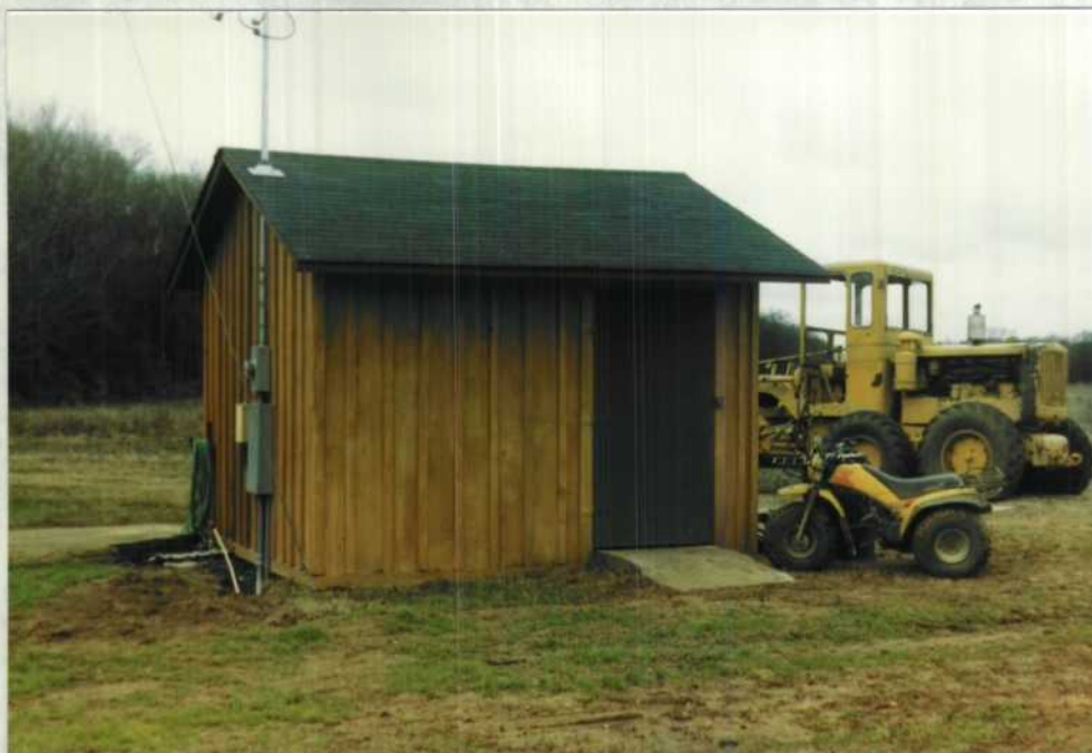
Fig. 12. The construction of a new 12'x12' cypress sided building provided much-needed storage space for tools and materials. 11/87 DME
