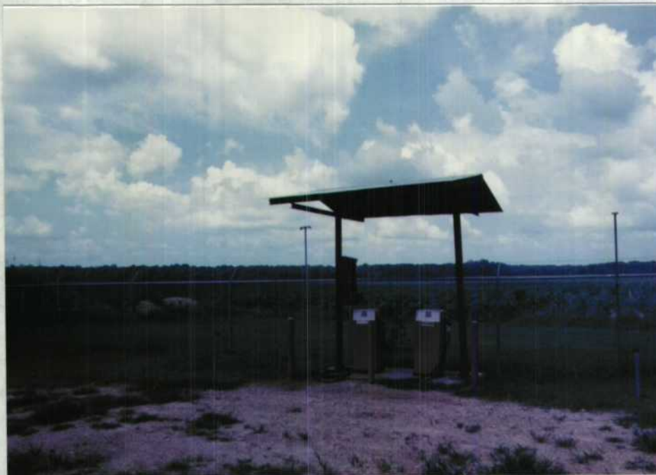
Fig. 8. Fuel station complete with safety bumper guards. 08/87 HWB
