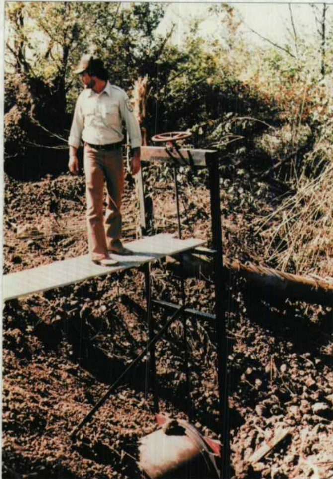
Fig. 34. Replacement of two deteriorated 12-inch pipes by a 36-inch and construction of a walkway were accomplished at the Silver Lake Impoundment.
