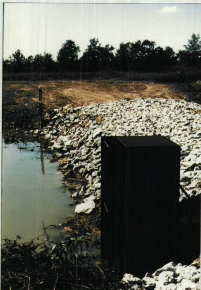
Fig. 16. This control structure, constructed near the mouth of Deep Bayou, created a 350-acre greentree reservoir. 08/87 TMW
