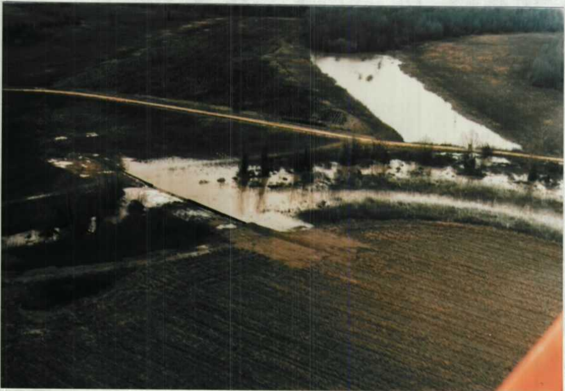
Fig. 12. Sheet piling structure.
