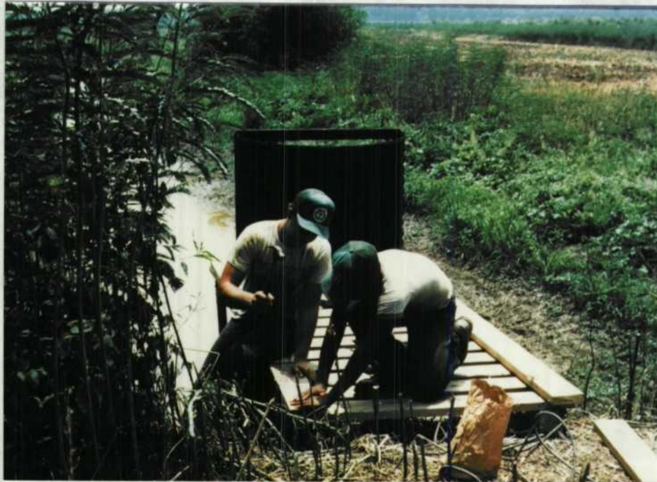
Fig. 14. Watch those fingers! YCC workers put the final touches on a walkway to the Open Ridge moist-soil unit control structure. 07/87 DME
