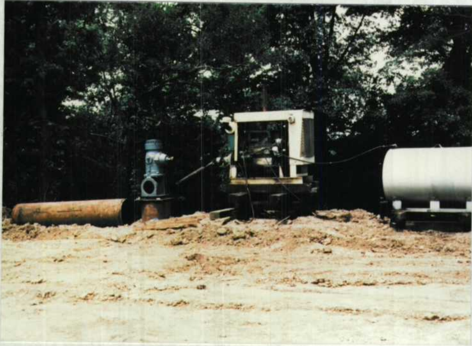
Fig. 31. A pump set in Silver Lake Bayou replaced a 100-foot irrigation well. 05/87 ALB
