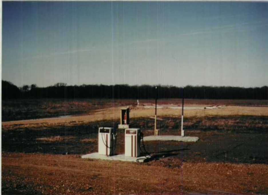
Fig. 17. A fuel station was installed at Gumbo Acres using new tanks and refurbished excess pumps. The concrete slab for the new shop building is in the background. 12/87 DME
