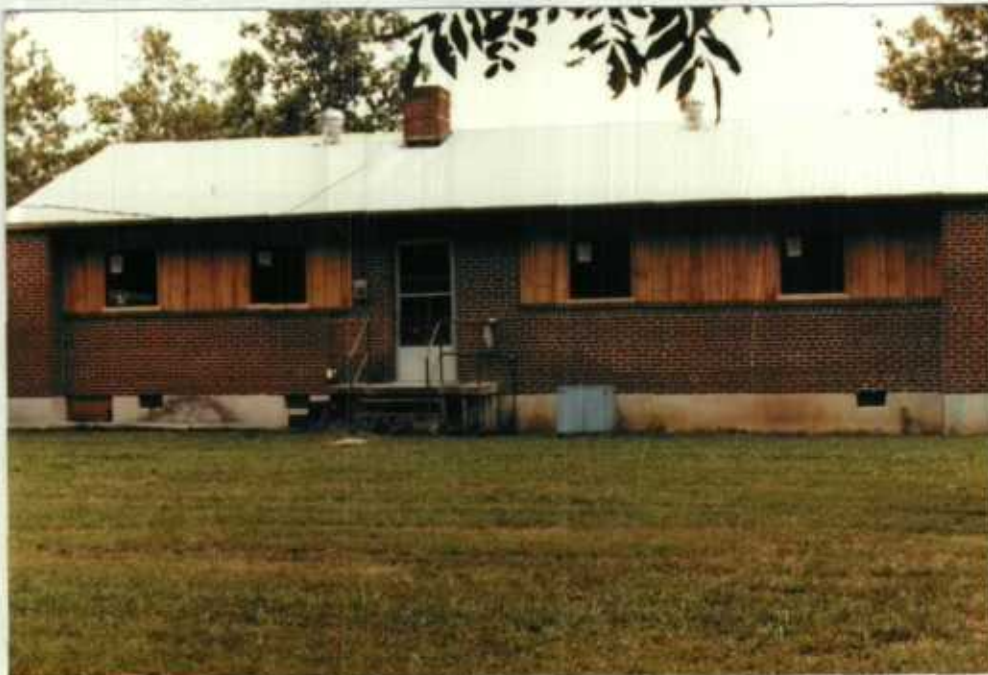
White shingles save air conditioning energy in summer. Smaller windows and insulation save energy both summer and winter. 12/82 TMW
