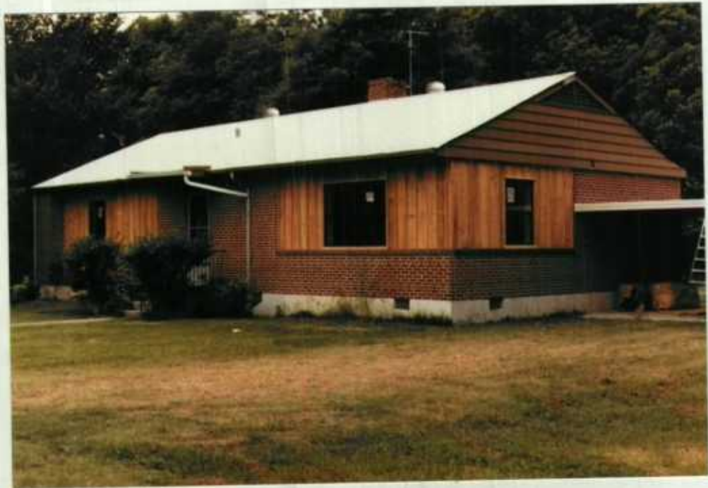
Quarters 22 after remodeling, thermopane windows are now 6% of the outside walls. 6/83 TMW
