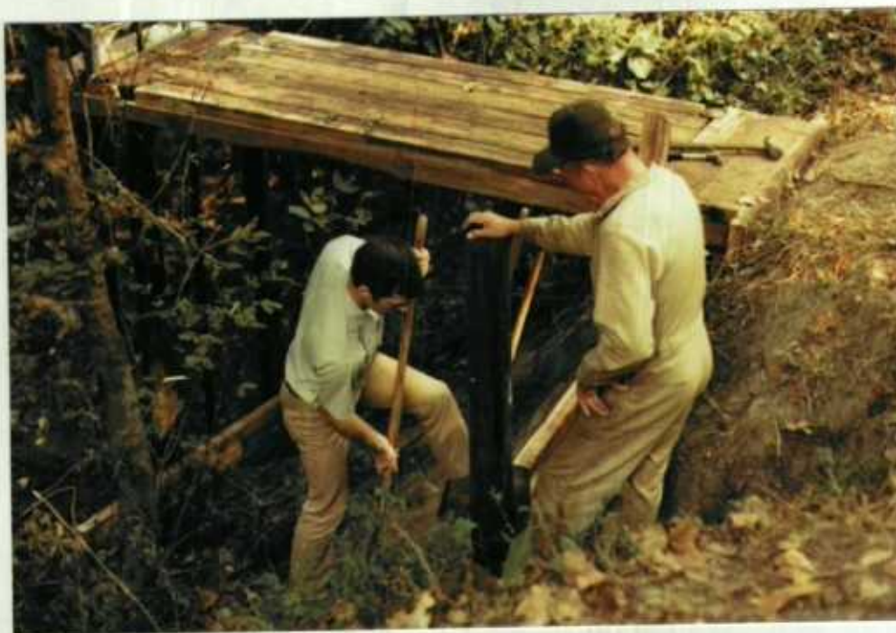
Lizard Lake walkway construction.
