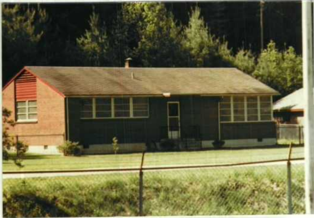
Typical R-4 house with hurricane windows on 29% of outside walls. 5/79 JTF
