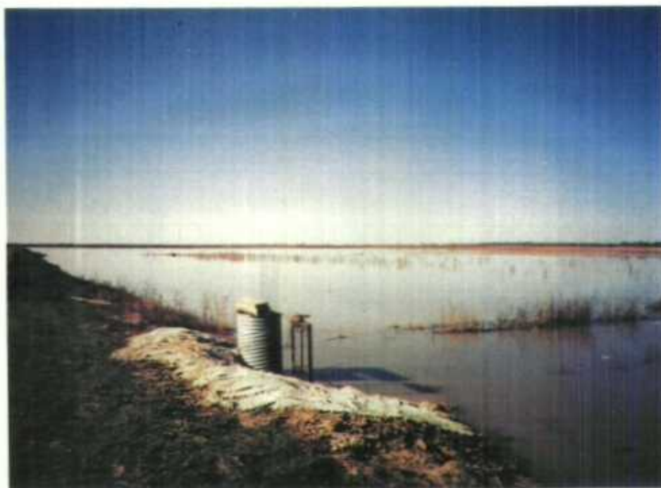
A one half mile levee built on an existing road dividing two impoundments. The levee and newly installed 24-inch screwgate and 42-inch flashboard riser allow flooding of 140 acre impoundment.
