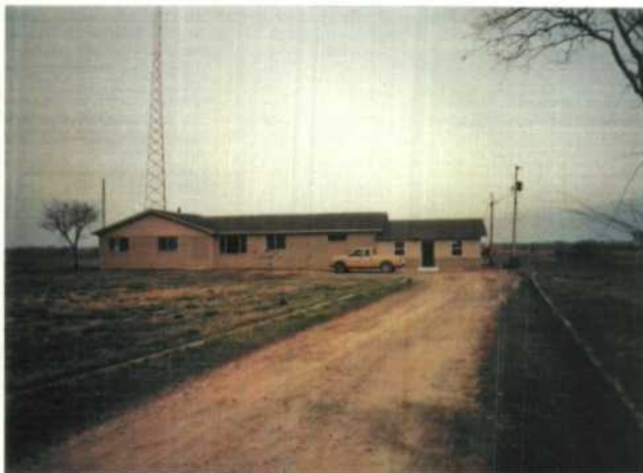
The new office, rehabilitated staff area and temporary living quarters at the Dixie Unit.
