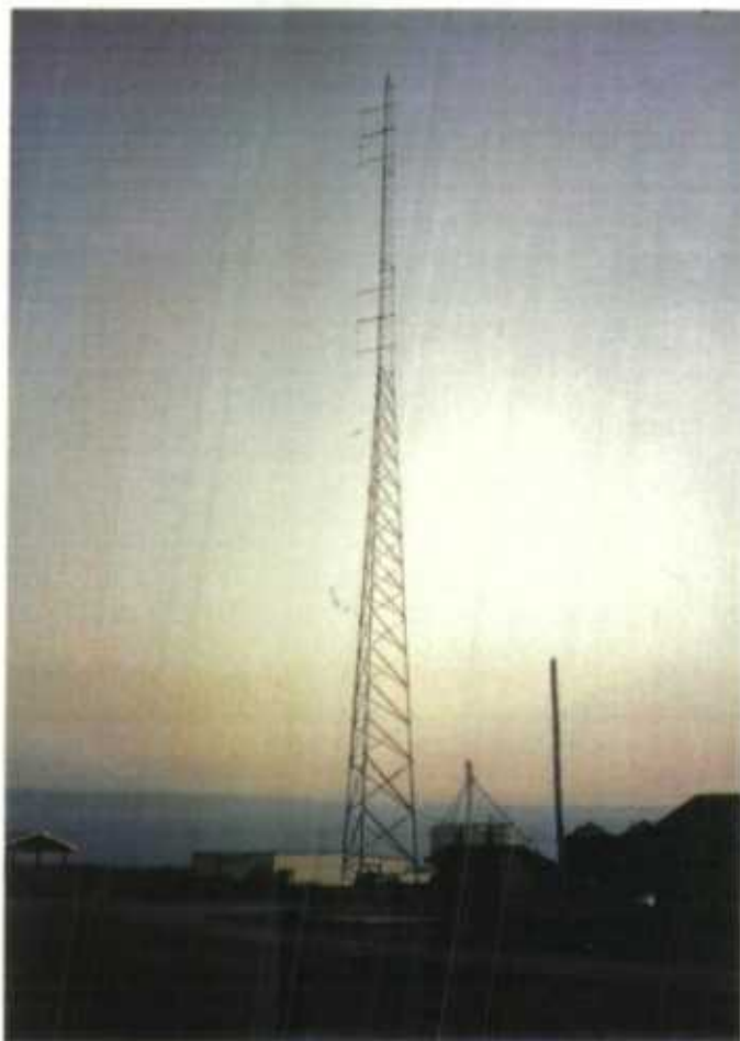
Free standing 140-foot radio tower at the Dixie Unit
