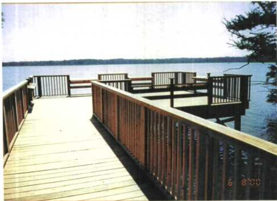
6/8/00 Print 00-1-21 GRM Completed Observation/Fishing Pier
