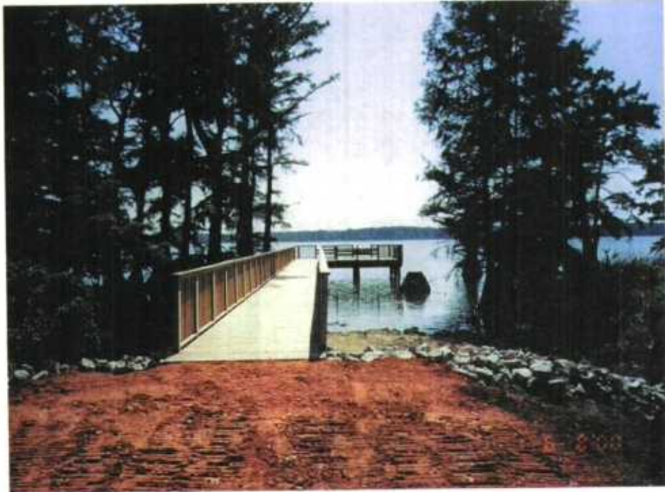
6/8/00 Print 00-1-19 GRM Completed Observation/Fishing Pier
