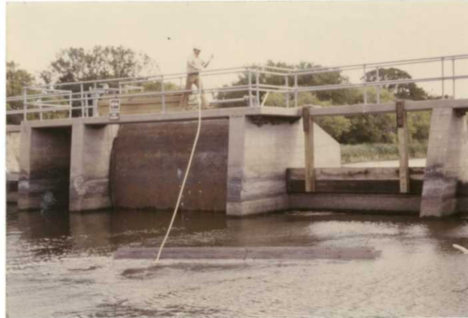
Figure 5. Four one-foot extension forms were floated downstream. (8-84-DL)
