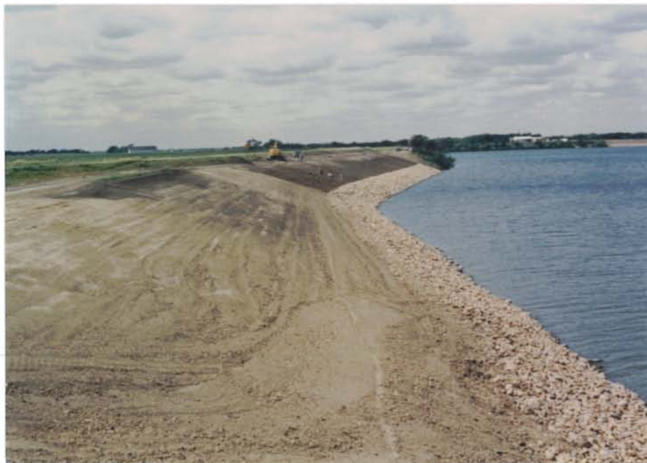
Riprapping on Lake Tewaukon to protect County Road #5 and the cemetery. WRH
