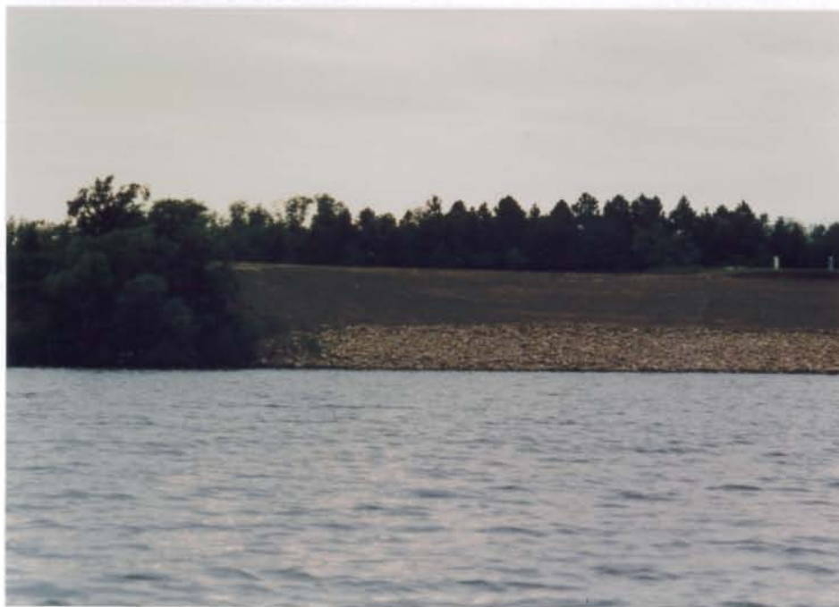
Riprapping on Lake Tewaukon to protect County Road #5 and the cemetery. WRH
