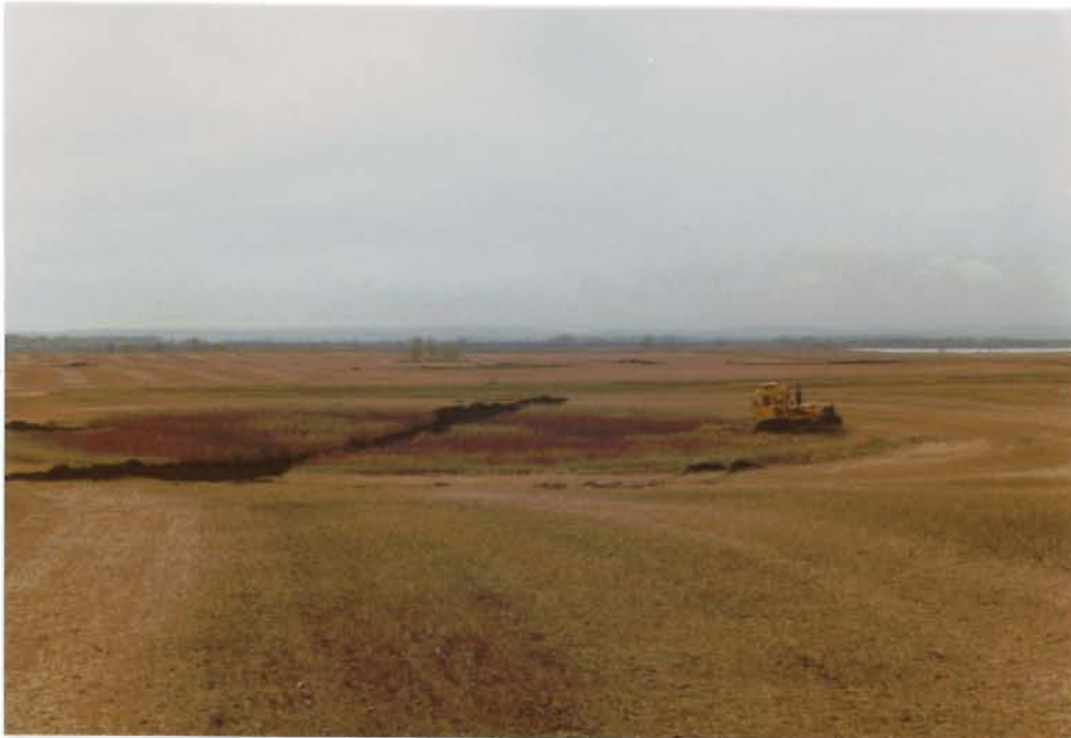
Mr. Berle Meyers and Sand Lake NWR's dozer worked a week cutting openings in vegetation choked wetlands. The spoil was pushed to the edges where it will be farmed in next spring. 10/83 - DGP
