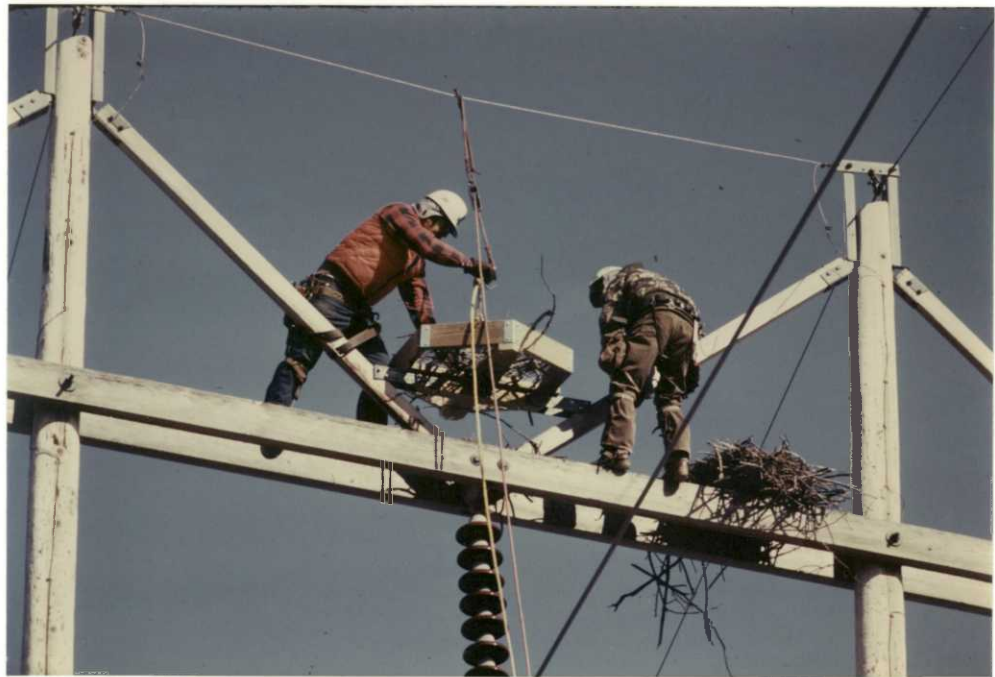
Preparing to bolt the platform in place.
