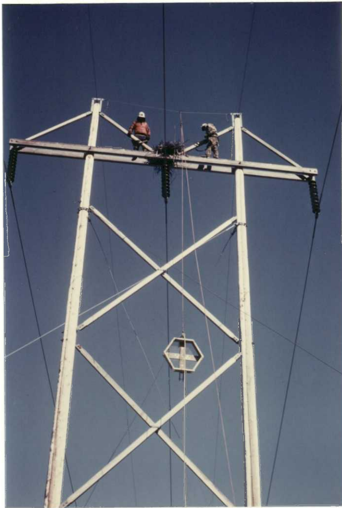
NSP crew hoisting the nest platform up the 75-foot tower.
