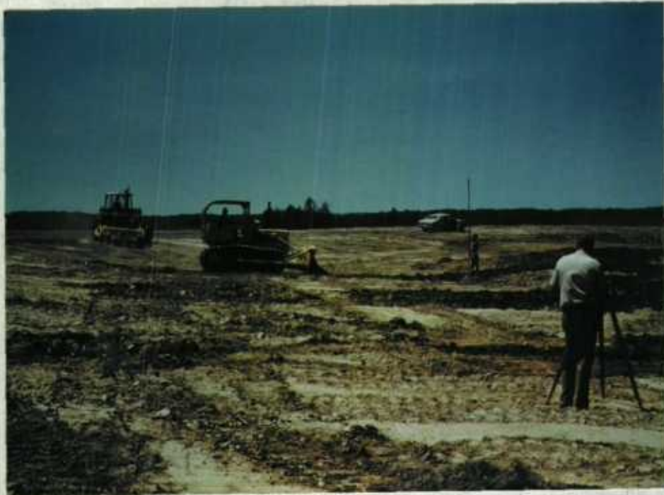
80-8-8. Soil Conservationist Eddie L. Reese "fine grades" all of the contours and drains on the entire Sulphur Well terracing project. (LR)
