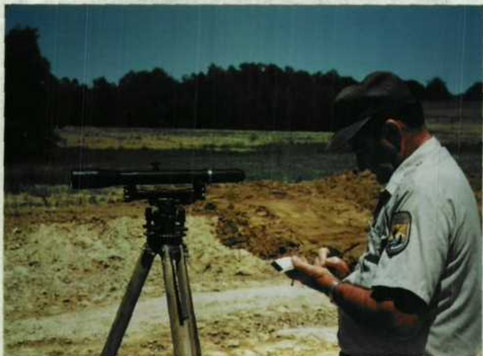
80-8-9. More than 7,000' of contour terraces were constructed on the Sulphur Well peninsula to help control water run-off and erosion. (LR).
