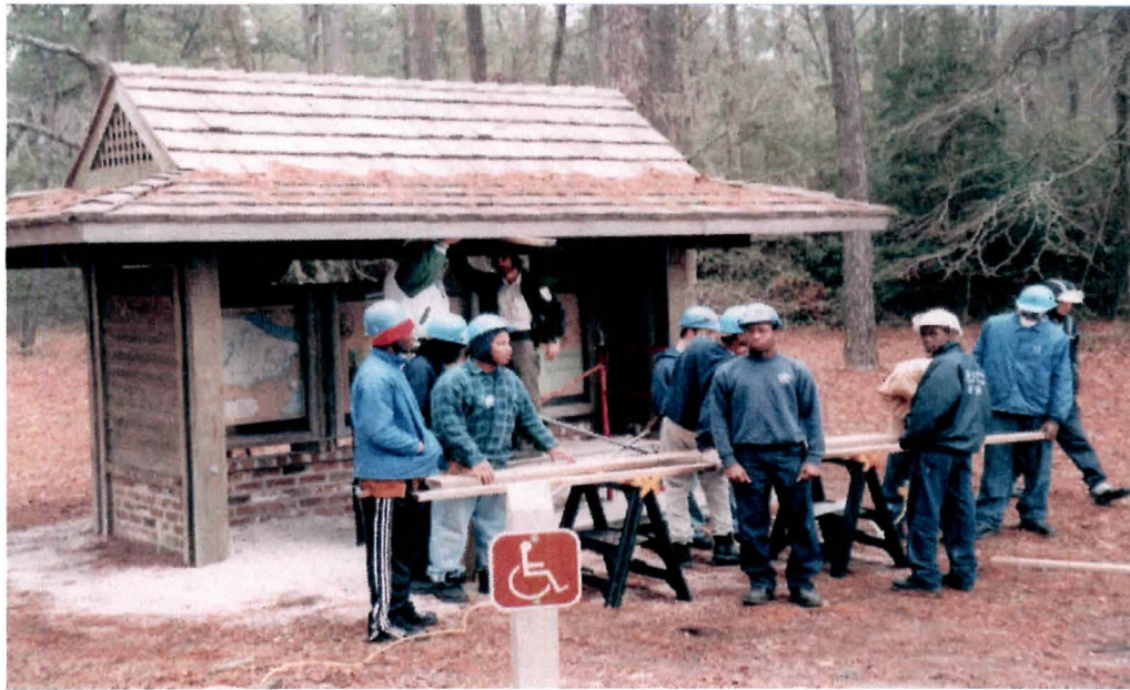
Job Corps workers completed repairs to the interpretive kiosk. (99-HSN5-PEM)
