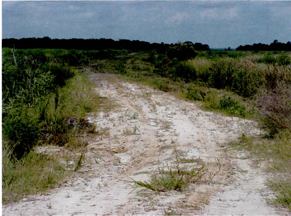
Results of Rehabilitation of Dike Separating Units 15 and 16. (99-SVH1-RW)
