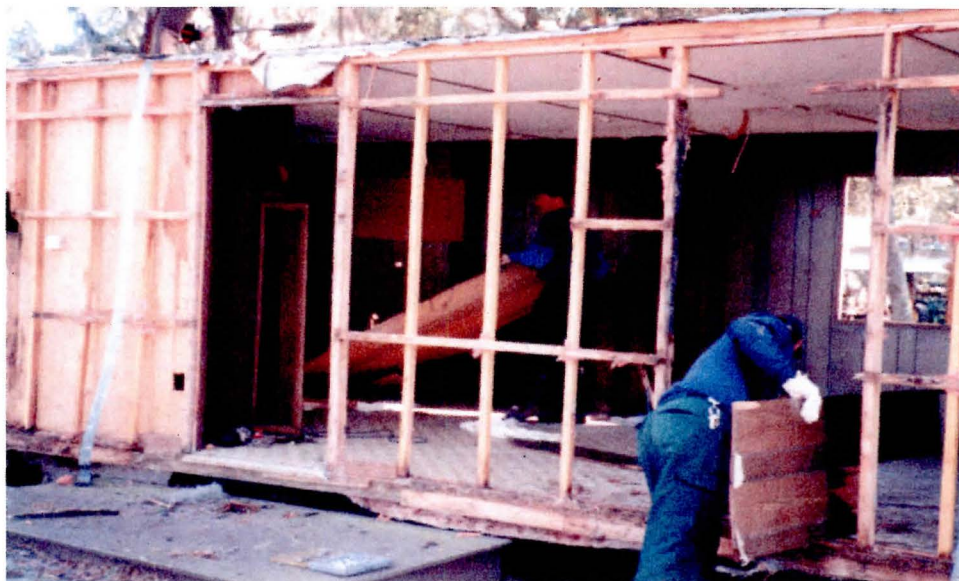
Firefighters and ROS Gilje dismantle the old staff trailer. (99-BLB3-SG)
