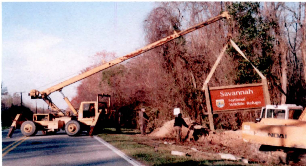
Post hole diggers were inadequate for this sign installation project. (99-SVH6-PEM)
