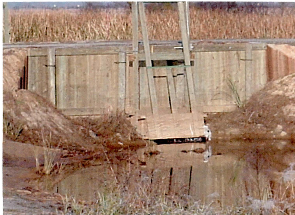
Rice field trunk installed in John Hill Canal. (99-SVH2-RW)
