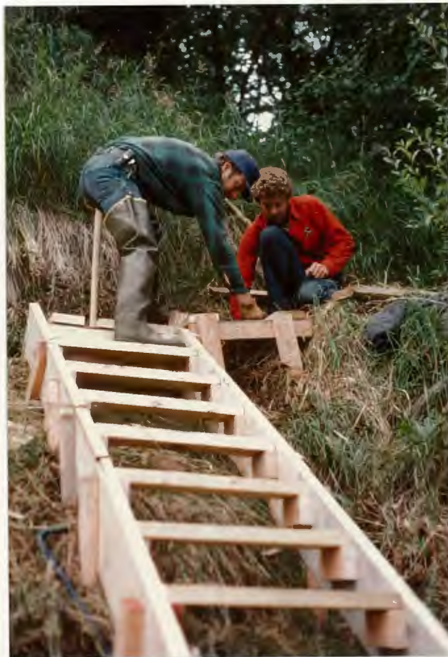
Fig. 43. Keeping on top of things with a little help from your friends...Manager Kent Hall and Volunteer Brad Engstrand designed, and with the help of other refuge staff, constructed a stairway from the refuge cabin down to the Selawik River landing.
