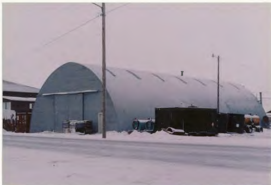
Fig. 40. Here is the Roger Nordlam quonset hut. A nice place to work when it's chilly outside! The refuge sub-leases 1000sq foot portion of the quonset with access to the heated shop, for $9000/year from the National Park Service.
