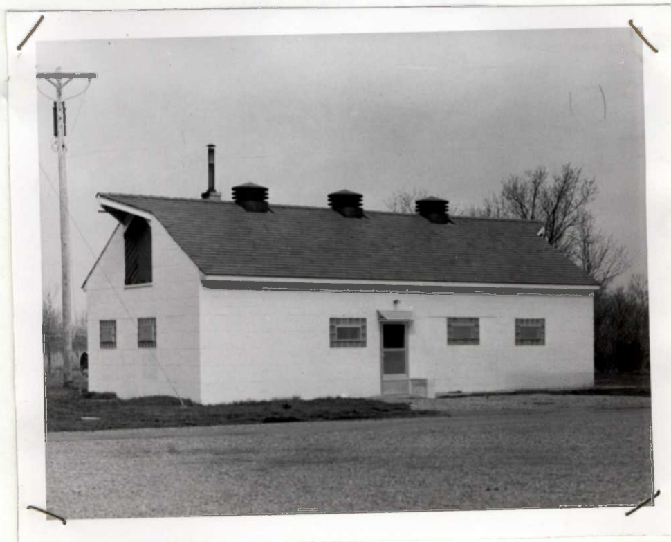
Transient quarters after renovation Exp. 394, 4/61, RRJ
