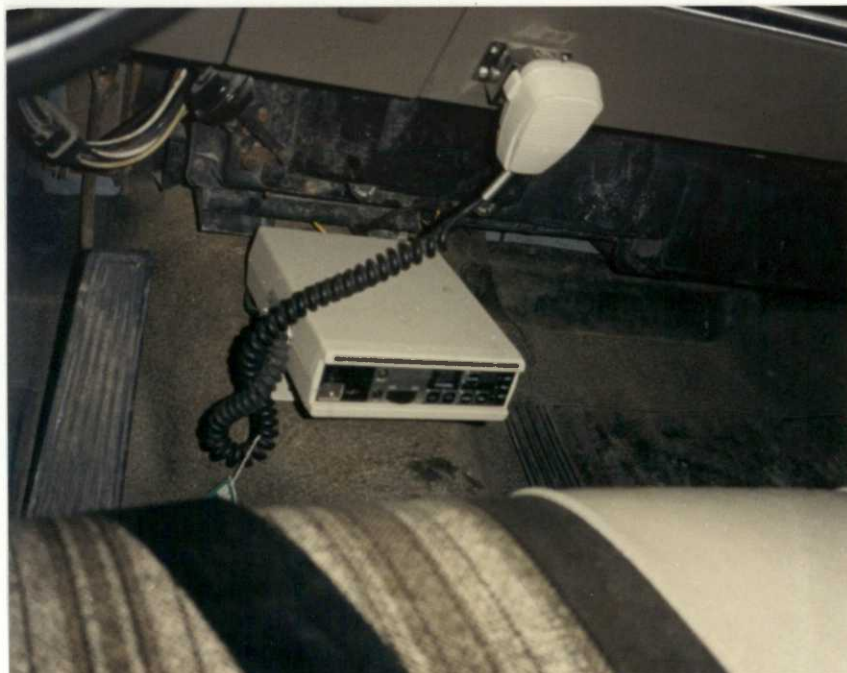
It took months to successfully debug the new radio system. (14MR86, R2-02, JI)
