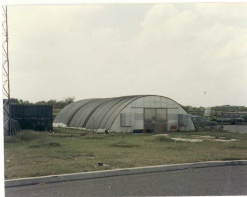
After -- The greenhouse is completed and in use. Its predecessor continues in use at the left, a shade structure consisting of shade cloth over a frame. (14MR86, R1-10, JI)
