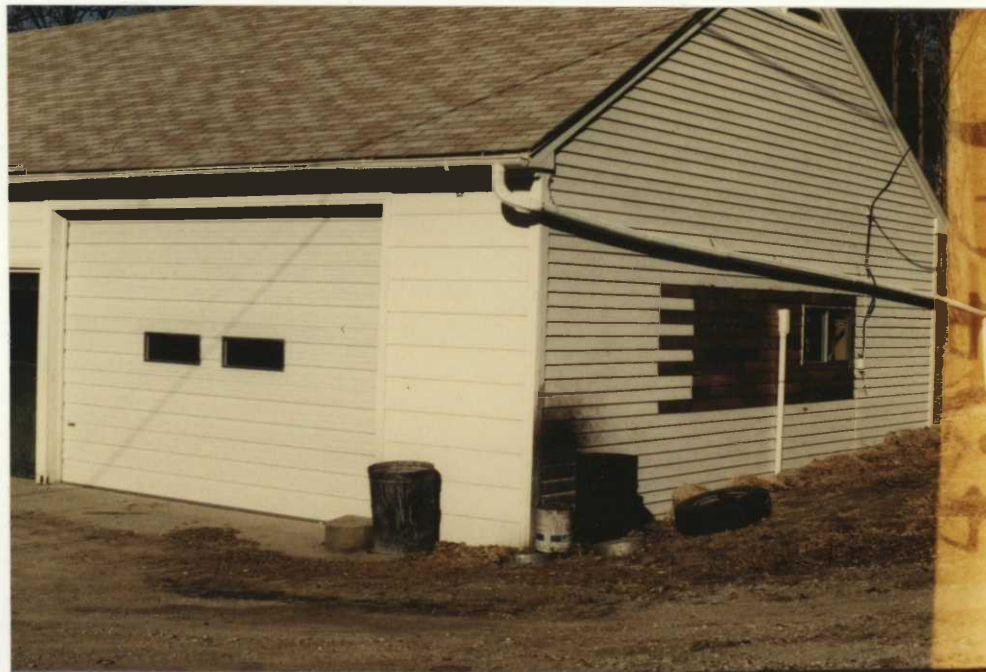
Refuge shop with new insulated door and window. 11/80 BAH
