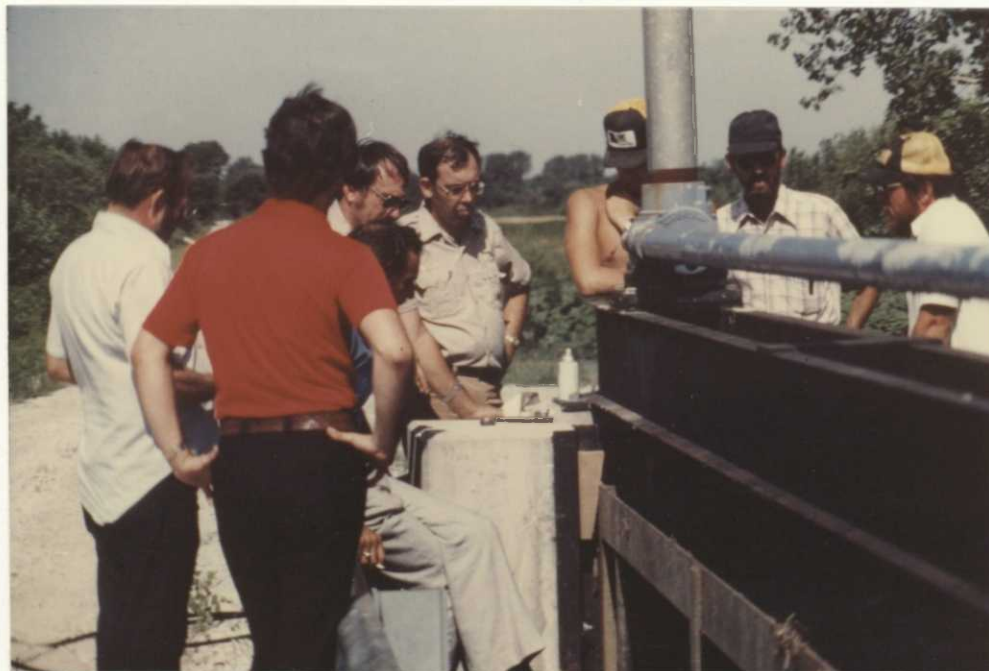
Meeting at the Squaw Creek roller gate. Represented are Armco Steel, Denver Engineering Center, Garney Construction and refuge staff. 9/80 JAG
