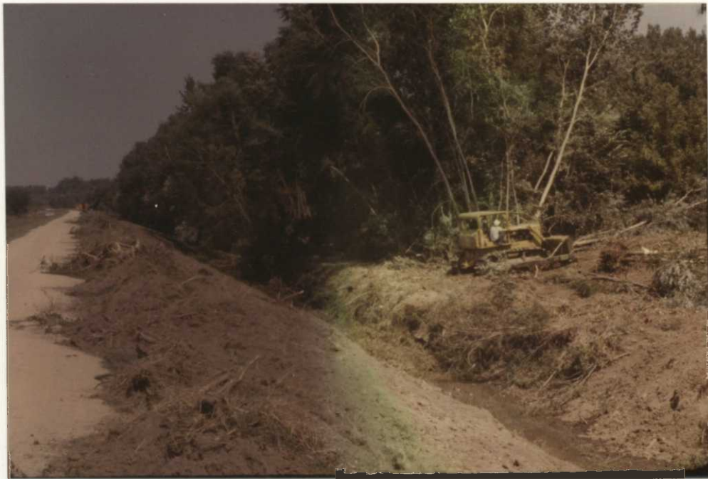
Clearing brush on Davis Creek ditch while awaiting settlement of conflicts with downstream landowners. 10/80 BAH
