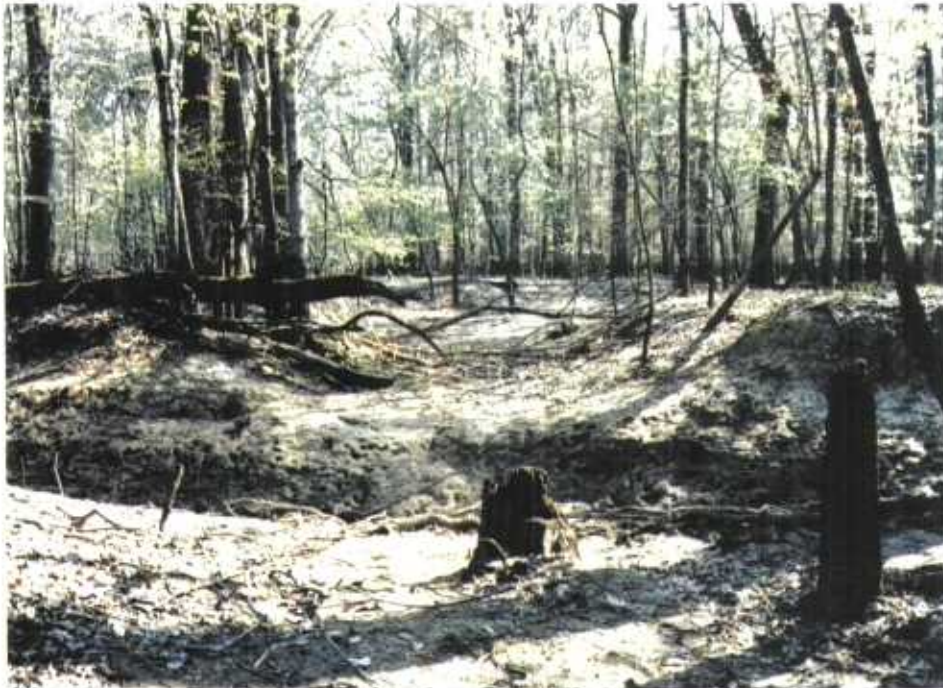
The Broadneck Swamp No. 1 man-made canal severed a few shallow drains that have historically drained the backslope of the natural river levee to the adjacent cypress-tupelo backswamp. 95-03-20 JLH
