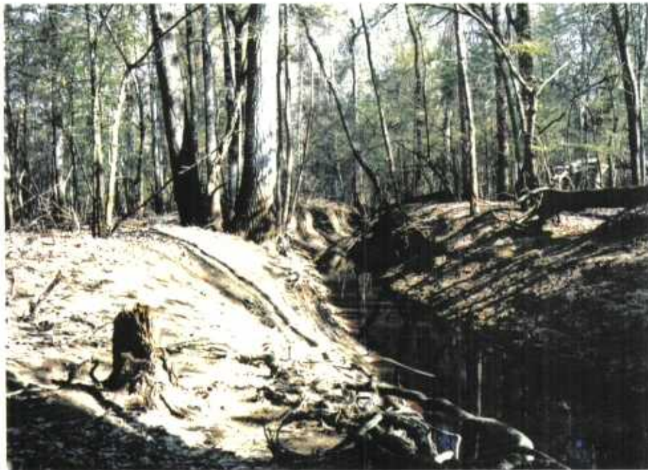
The canal's depth, here approximately eight (8) feet, allows rapid flushing and draining of the adjacent cypress-tupelo backswamp. 95-03-21 JLH
