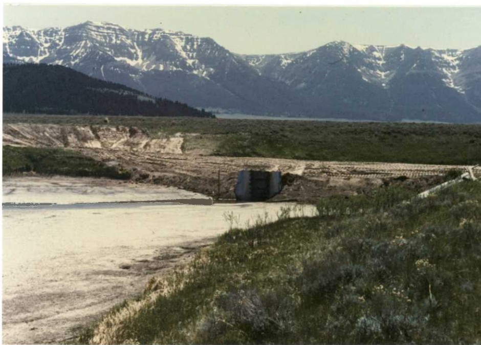
Revamped dike at Culver Pond
