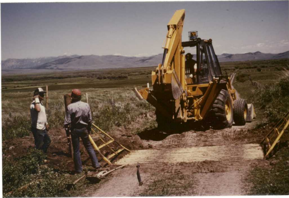
Maintenance crew installing cattle guard on road to airport. One-half mile of fence was removed and the guard reset during this project. BR
