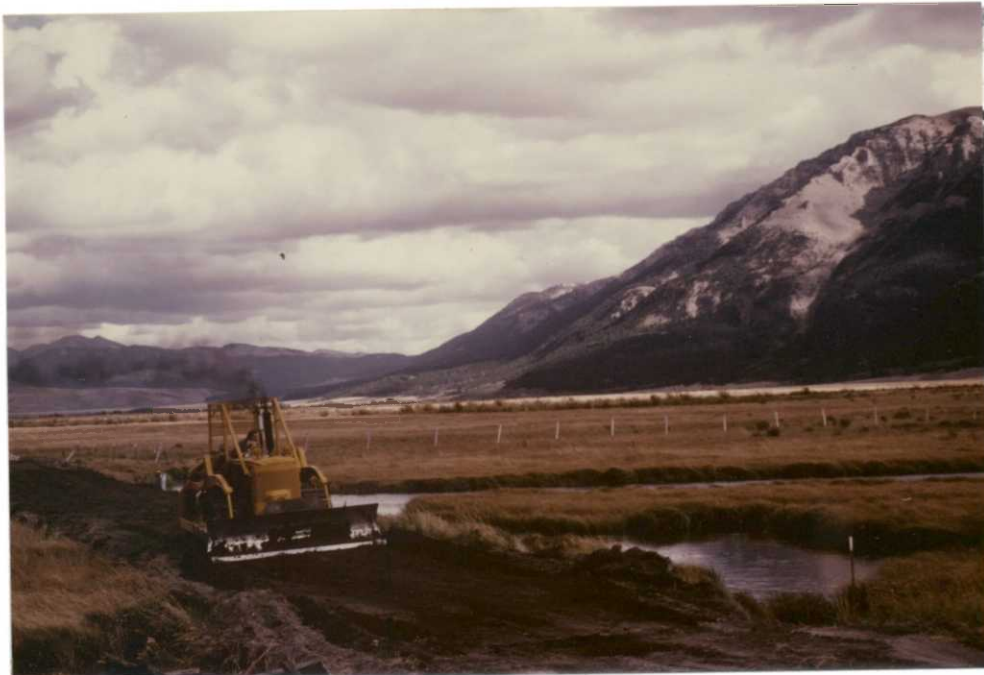
Young rebuilding dike on Cole Creek Slough.
