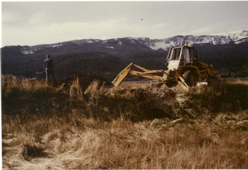
Maintenance crew installing culvert in Sparrow Rond to facilitate drawdown. BR
