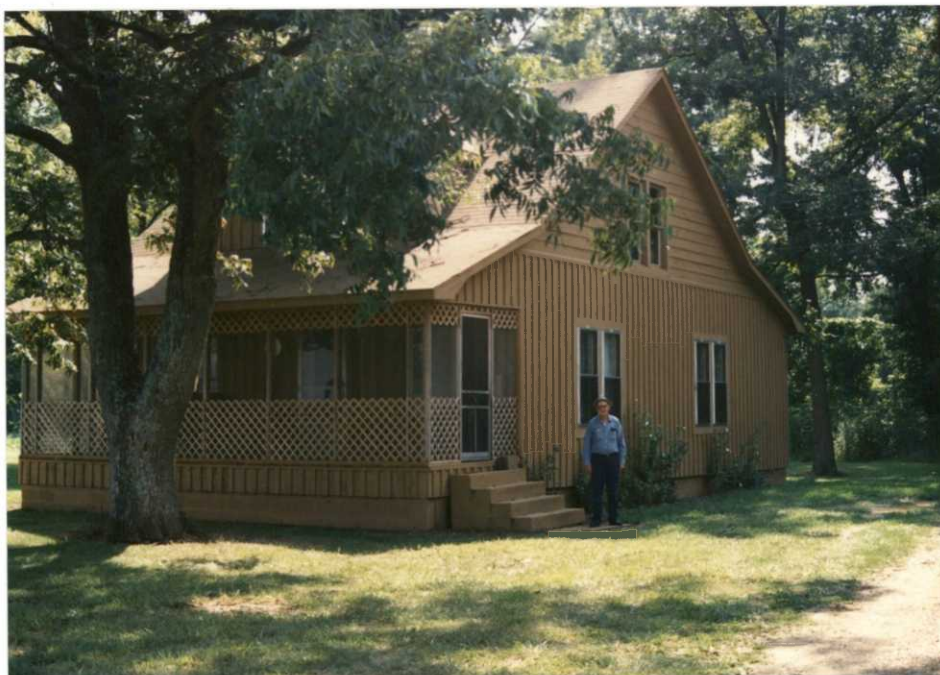
Long Point residence after application of exterior stain. 8/90 GHS
