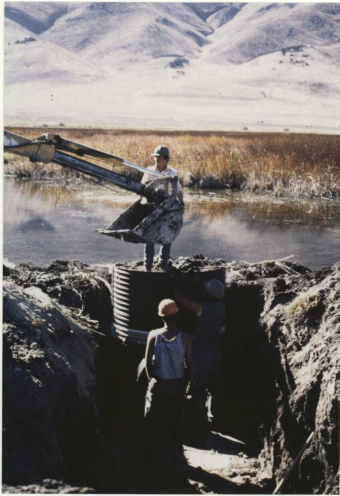
Figure 14. Installation of water control structure by Art Lacey Construction. SMB 09/87
