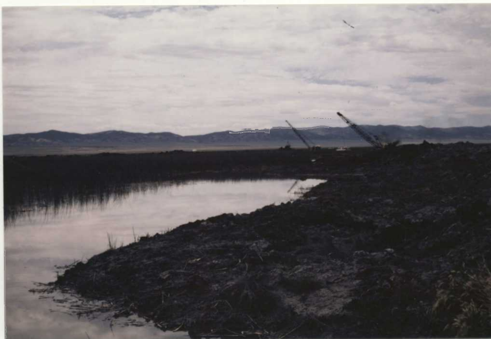
Figure 11. Completed channel in the southwest corner of the East Sump. SMB 07/87
