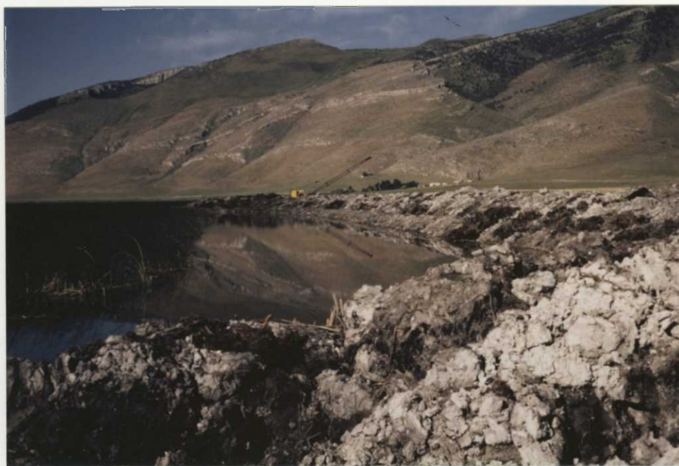
Figure 13. Cleaned channel in the northwest corner of the East Sump. Material from this channel and the dredged channel on the opposite side of the dike completely covered this dike to depths of six feet - a real challenge to spread and blend into the surrounding dike system. SMB 06/87
