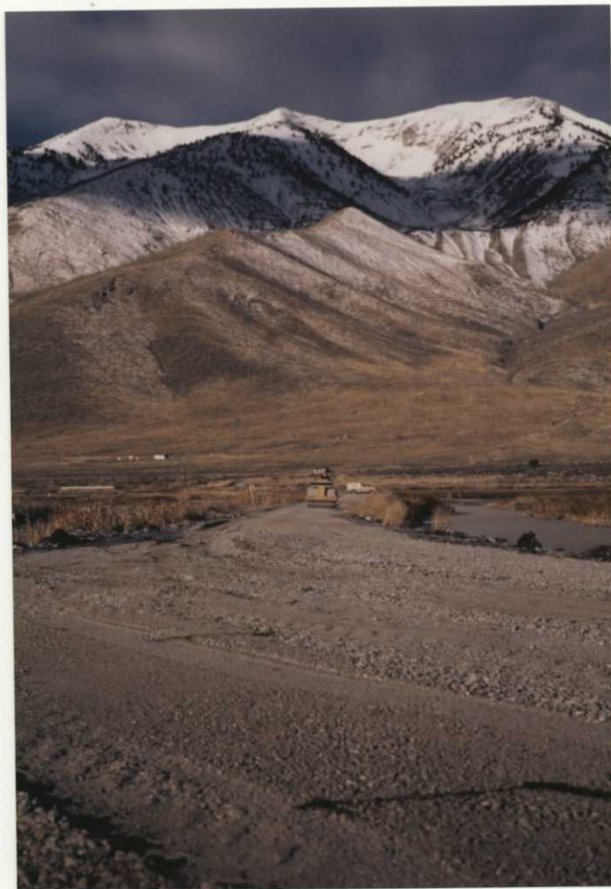
Figure 28. Final compaction of the crushed rock greatly improved the roads. This picture was taken at approximately the same location as Figure 25. SMB 12/87
