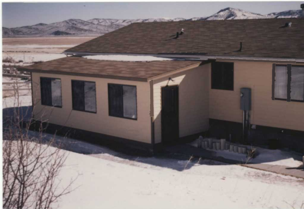
Figure 23. Newly built rear entranceway on Quarters 101.
