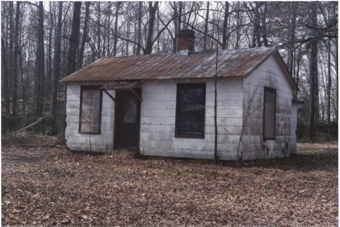
"James River NWR Manager's House" Old hunt club house slated for demolition.
