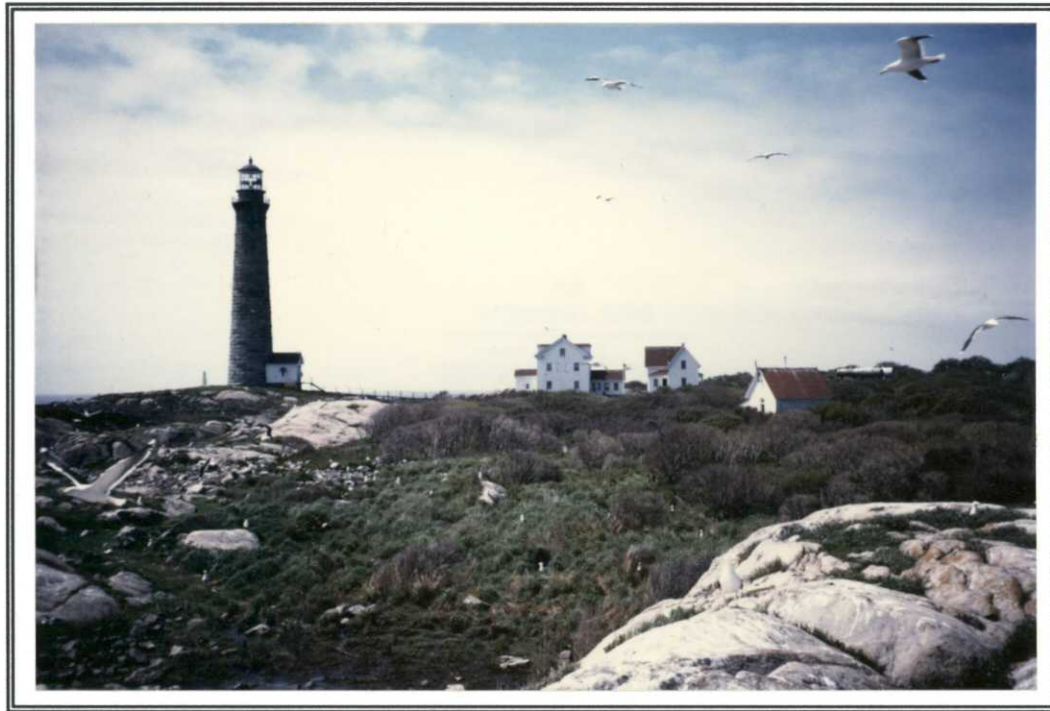
The North Tower at Thacher Island NWR (Nakai, 5/94)
