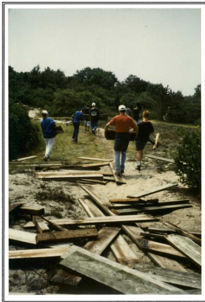
Turning Point, Inc. helped out on boardwalk construction by carrying out old sections of boardwalk.
