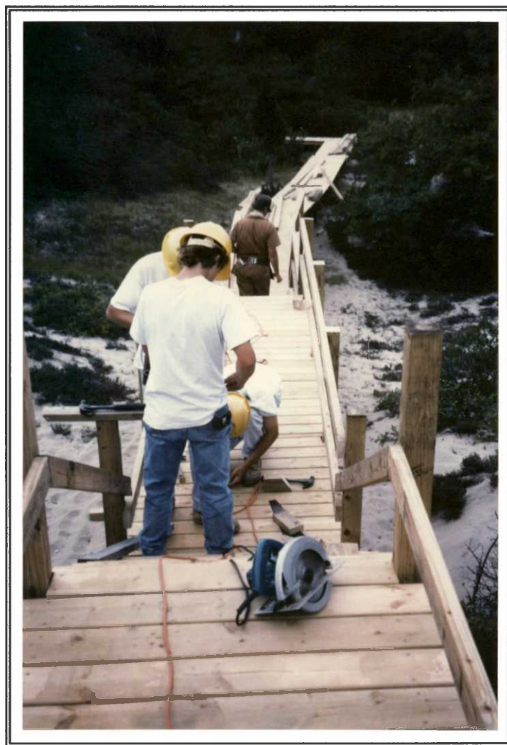
Constructing the new section of boardwalk at the Dune Loop (Fraser, 7/94)
