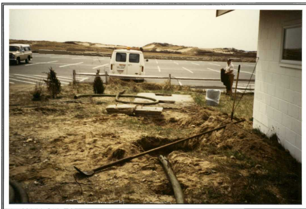
Plumbing repairs at the VCS included new lines, a new vault pump and a pump out of the holding tank. (Burke, 5/94)
