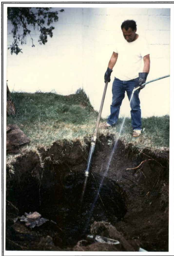
A new septic system was installed at the Headquarters building this year. (Drauszewski, 10/94)
