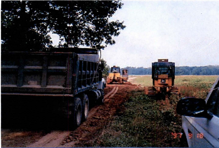
Dike Construction at Griffin Low-Grounds
